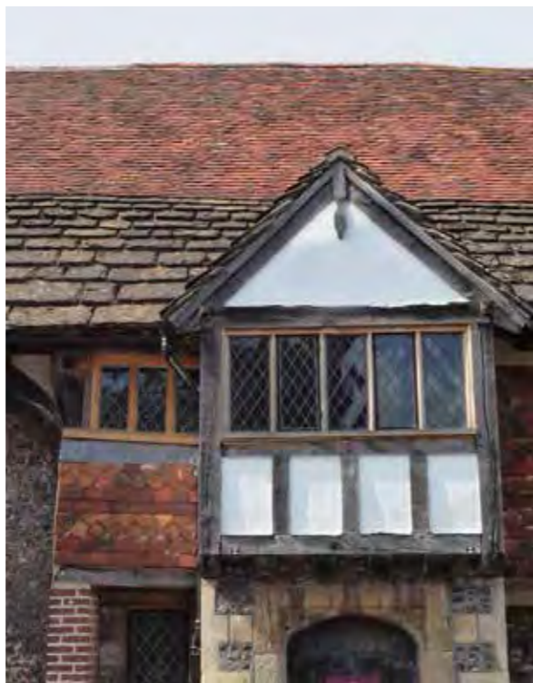
LEFT Horsham slate and clay tiles CREDIT: SPAB
