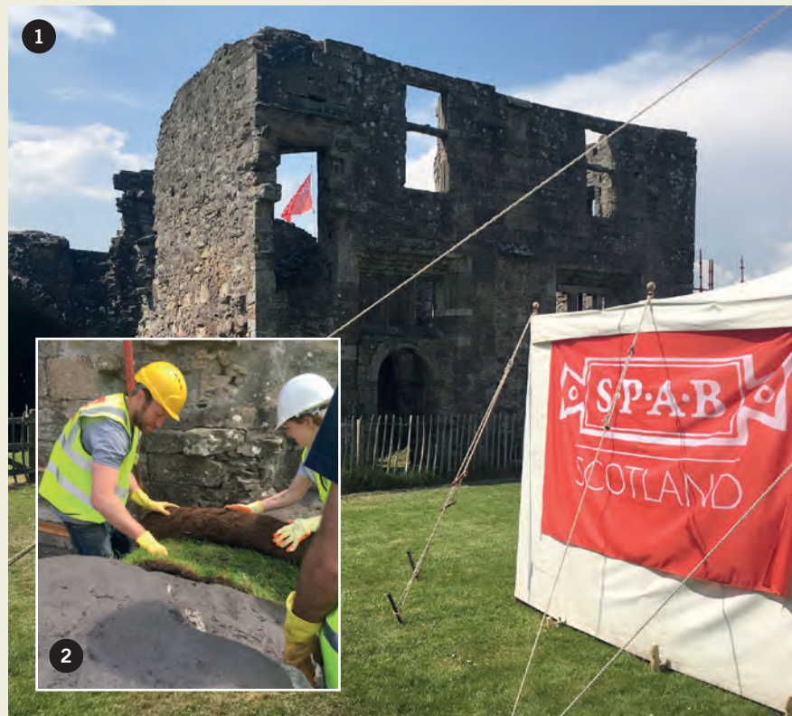
2 Turf being laid on Balmerino Abbey’s wall head, as part of the soft capping process (SPAB)
