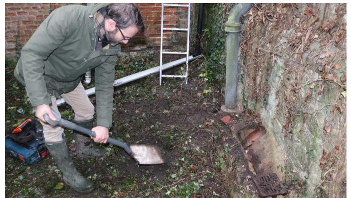
Matthew Slocombe carrying out exploratory work to investigate drainage. November 2019
