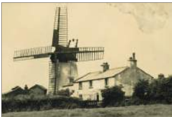
1940s Great Singleton, with all sails in tact, but minus the fan. The mill was at this point run by gas engine.
