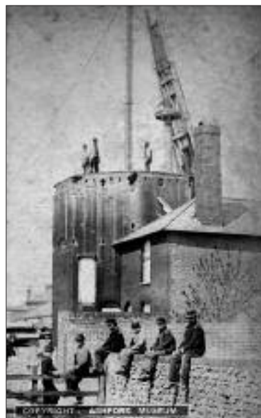
Fig. 3: Dismantling at an advanced stage.
