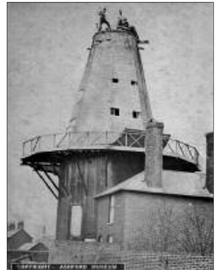
Fig. 2: Dismantling Regent's Place Mill.
