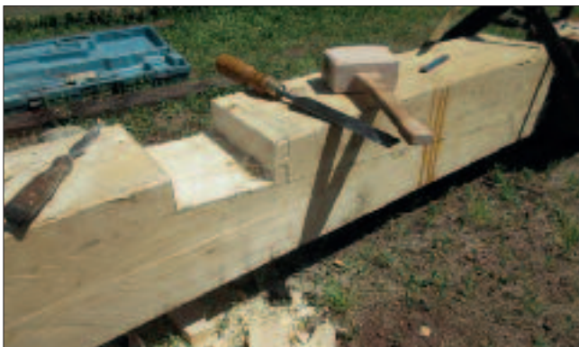
Scarf marked out, many downward cuts then the offcut chiselled off, then more. I cut the second one 33 times over the 900mm overlap.
