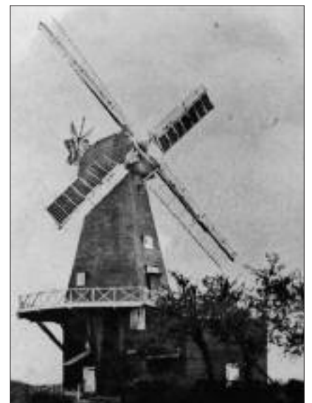
Fig. 4: Regent's Place Mill as rebuilt at Boundsgate Corner, Badlesmere.
