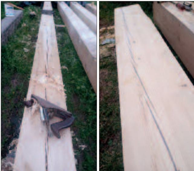
Filling the 'sbakes' in the spruce beams for the stretchers with epoxy resin.
