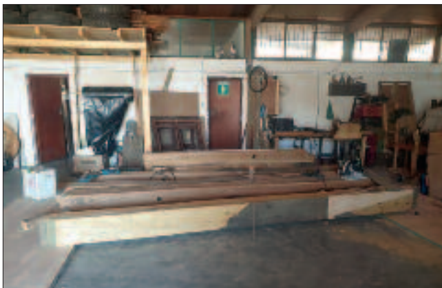
Jon has been busy lengthening the Bilinga beams for the sheers.
