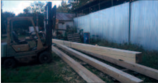
Selecting the straightest pair of spruce beams for the long stretcher.
