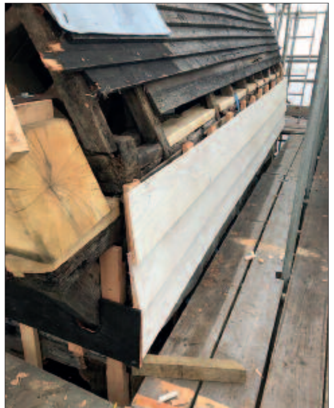
New weatherboarding going on. Picture – Dorothea Restorations.
