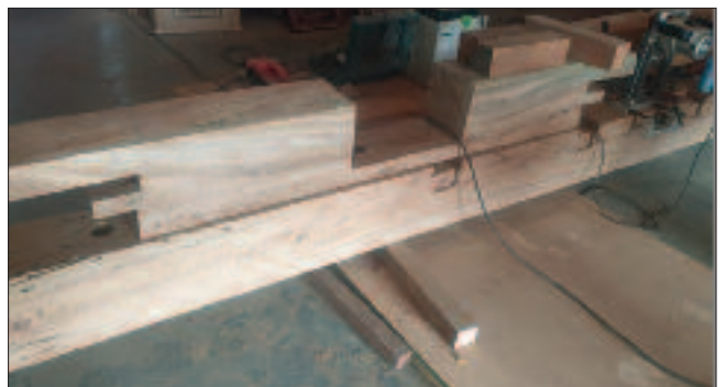
The beginnings of the tail beam, which will be beefed up, back and underneath.
