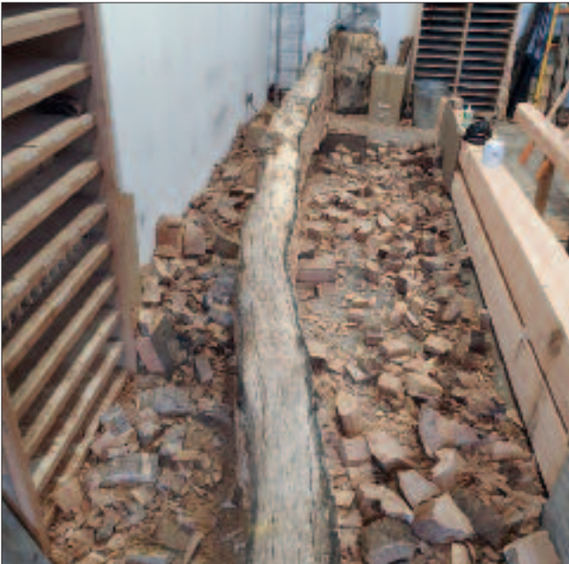
Timber for the new tail pole. Picture – Dorothea Restorations.
