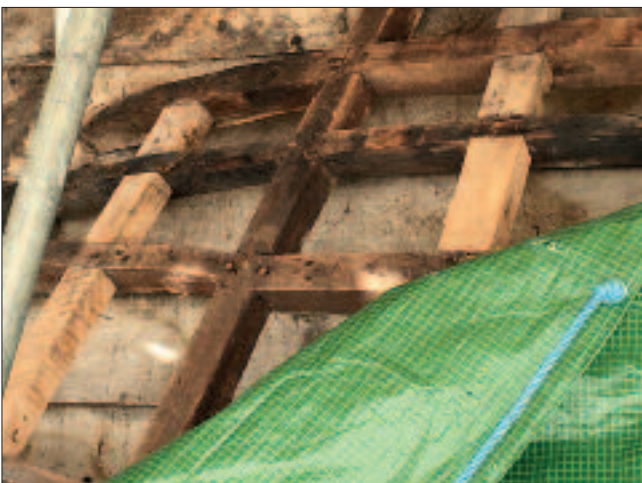
Timber repairs to roof of the roundhouse. Picture – Mildred Cookson.
