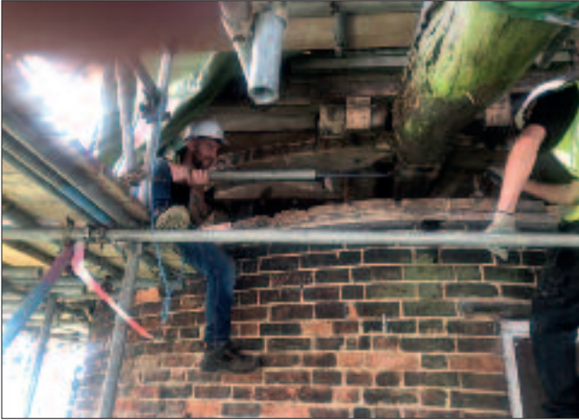
Removing the old tail pole. Picture – Dorothea Restorations.
