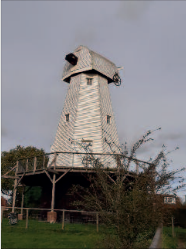
Woodchurch Windmill without sails or fantail following damage by high winds in 2019. Pictures – Carole Leith.
