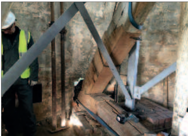
Quarter bar and cross-tree repair. Picture – Mildred Cookson.
