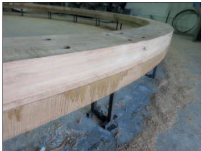
The curb ring after sizing.
