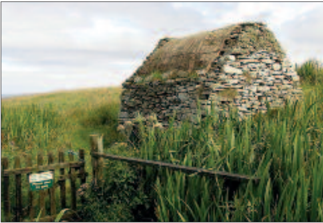
Fig. 3. The restored Southvoe Mill on the Burn of Wiltrow at the Croft House Museum, Southvoe, Dunrossness in 2007. Picture courtesy of Robbie Work.
