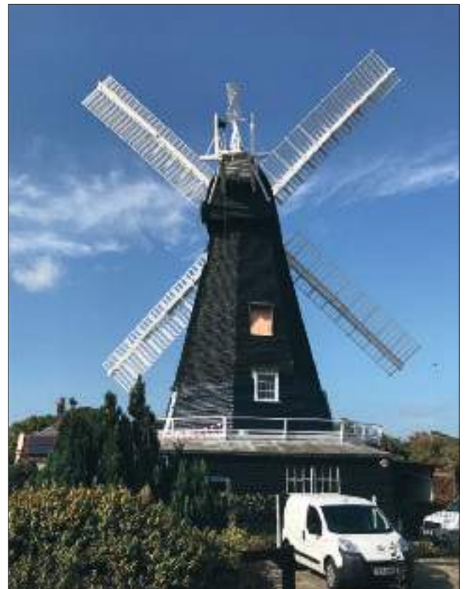
Tarring and window repairs being carried out by Owlsworth IJP at Drapers Mill, Margate in September 2019.
