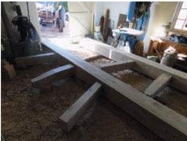
New sheers, test fitting new puncheons.
