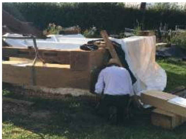
Fitting new weather beam onto cap frame (cap frame being upside down at this stage).
