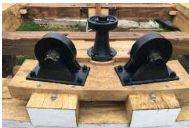
Weatherbeam truckwheel and centring wheel assemblies.
