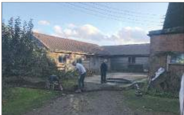
Electricity supply to West Kingsdown Mill being relocated underground by IAC Ltd in November 2019.
