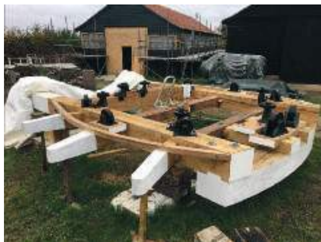
Cap frame with overhauled running gear in position.
