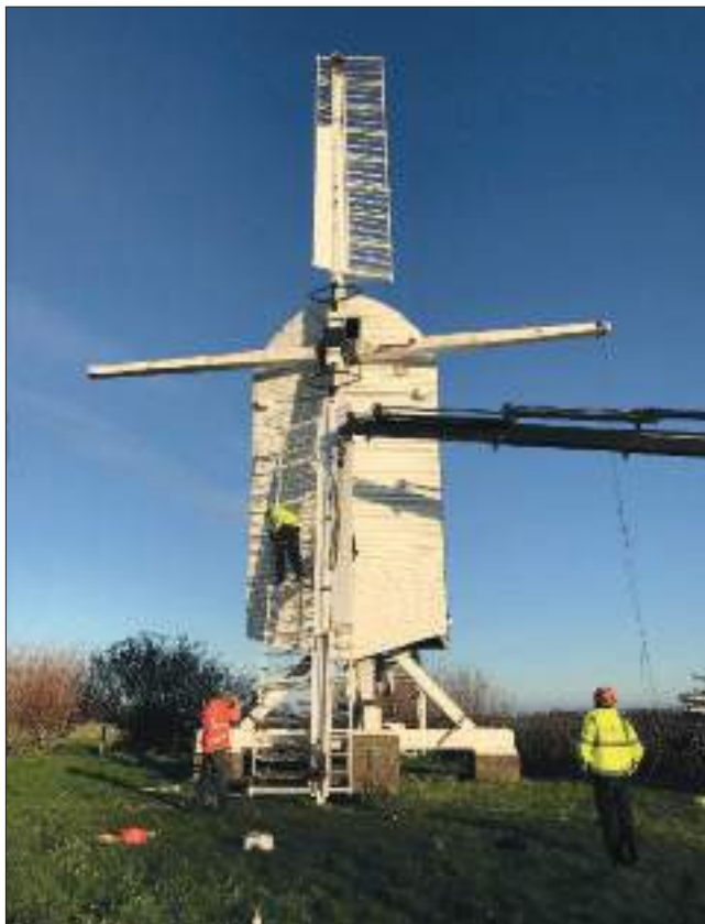
Sweeps being removed for repair and repainting by Tim Whiting at Chillenden Mill in December 2019.
