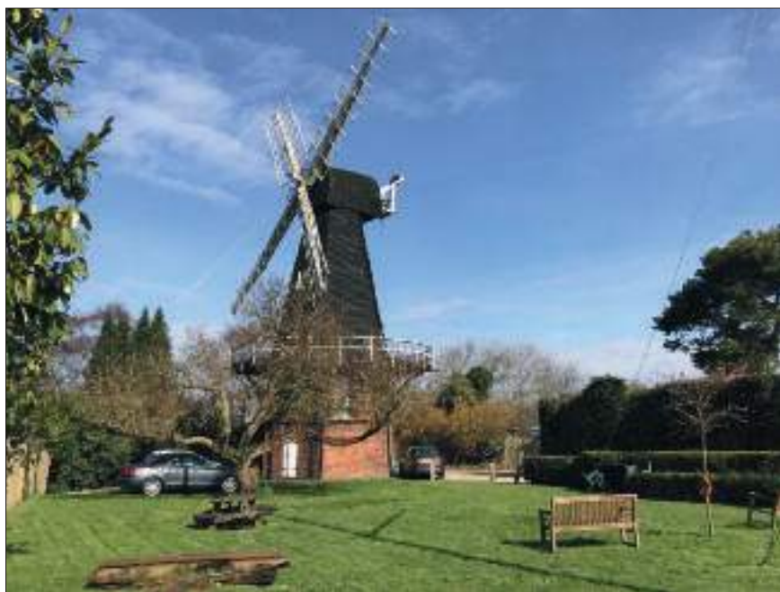
Meopham dismantled 2018 – Meopham Mill in 2018 with fantail blades and sweep shutters removed for safety.
