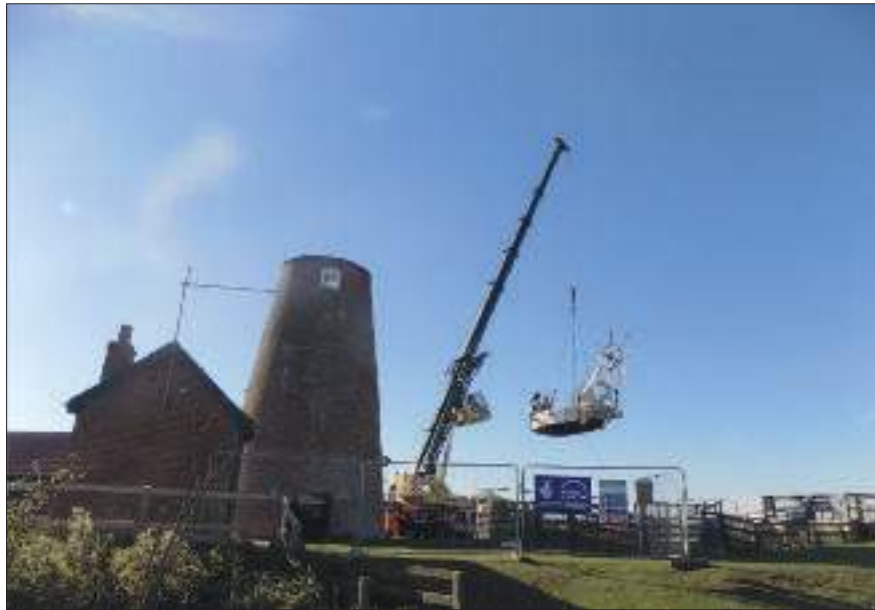
October 2018 – lifting off the cap frame
