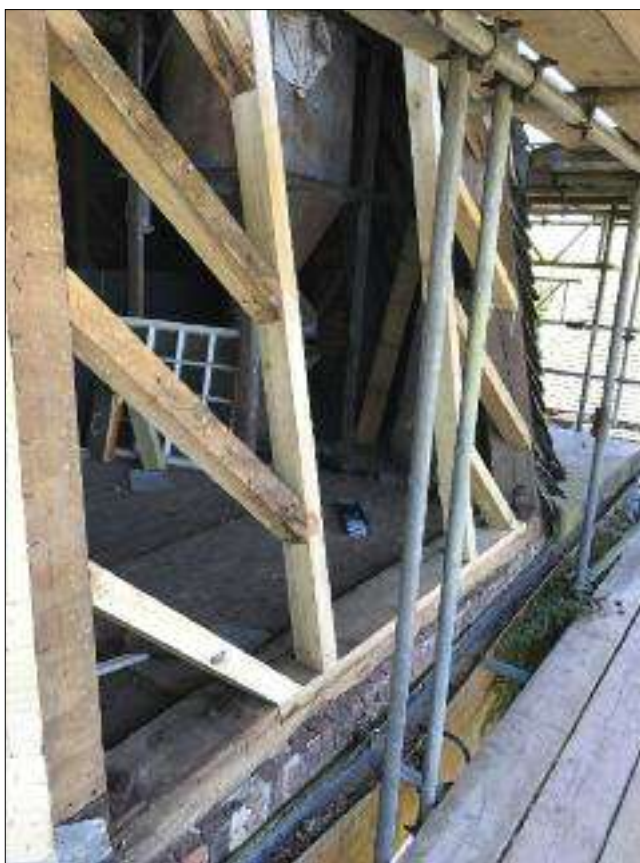
Repaired framing at meal floor level, West Kingsdown Windmill. Picture – Luke Bonwick.
