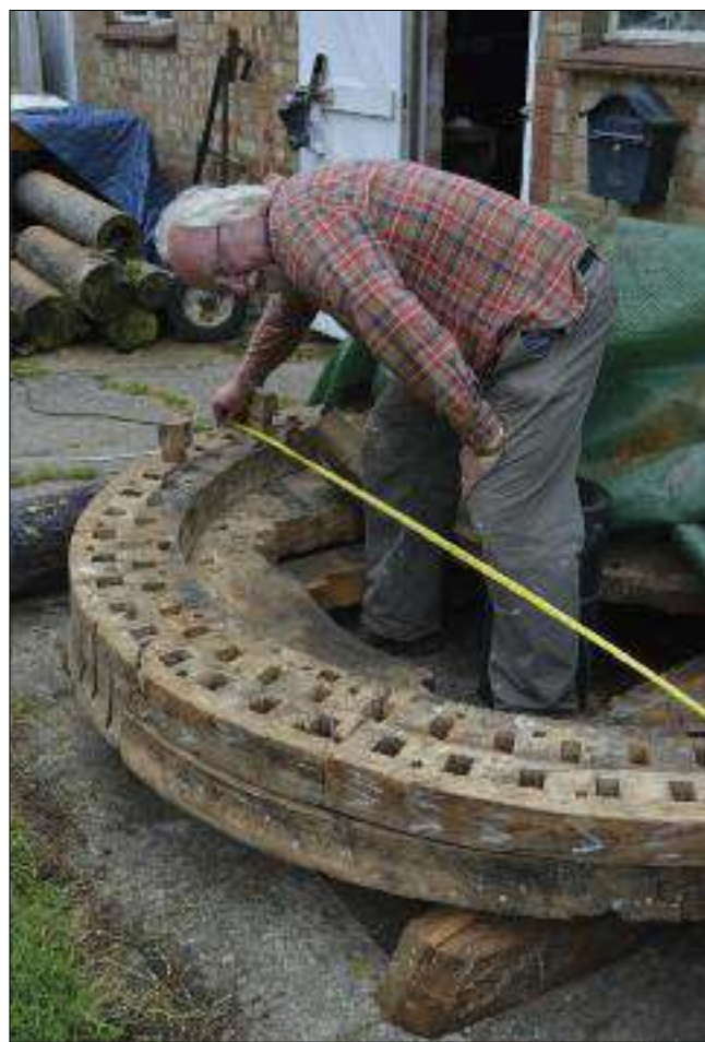
Dave Pearce, millwright at Wicken Windmill, measuring up the Great Gransden brake wheel.
