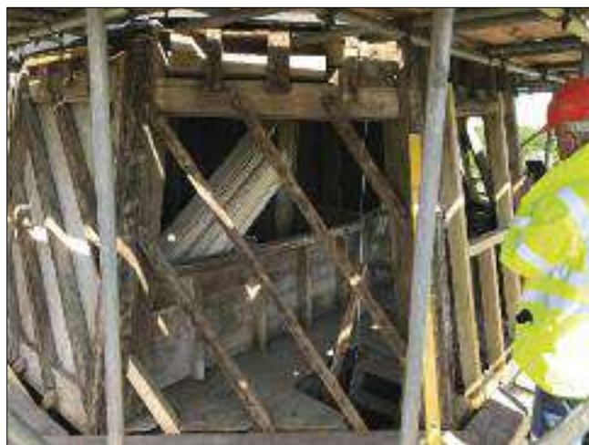
Councillor Michael Payne inspects the exposed bin floor wall framing of West Kingsdown Windmill. Picture – Luke Bonwick.
