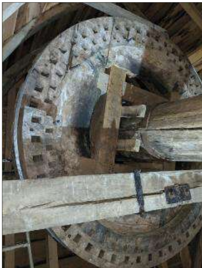
The Great Gransden brake wheel during the refitting of the elm felloes and showing the arrangement of oak spokes and elm slabs.
