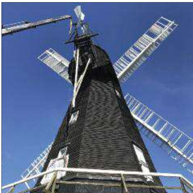
Removing the fantail from Herne Windmill. Picture – Tim Whiting.
