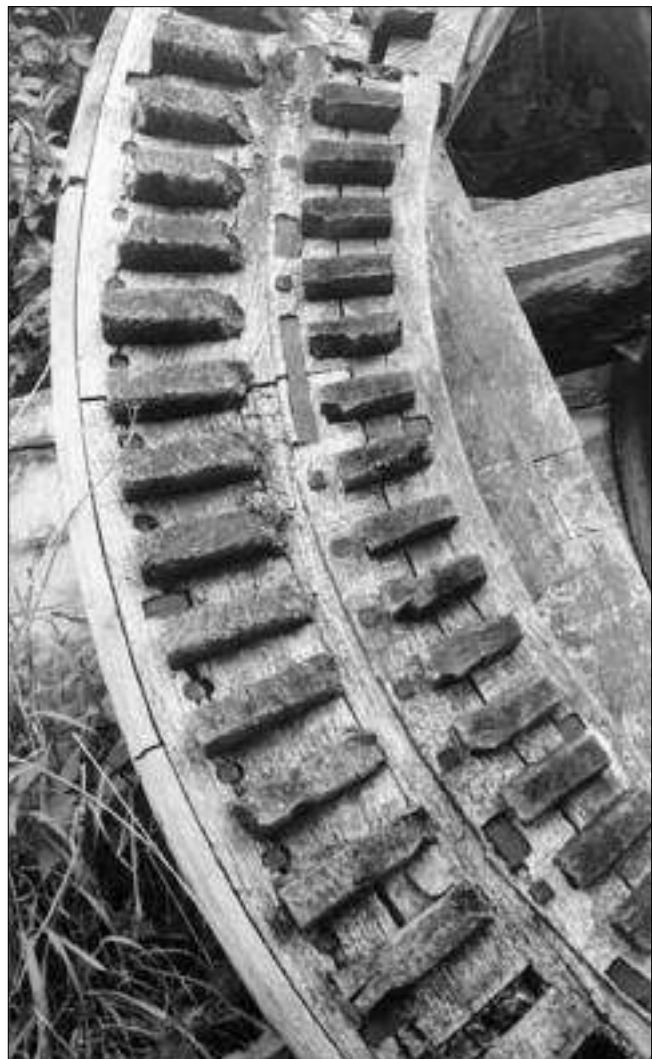
Brake wheel from Mortimer's Mill, Eye in September 1960. Picture – Ken Farries Collection, © Mills Archive Trust.
