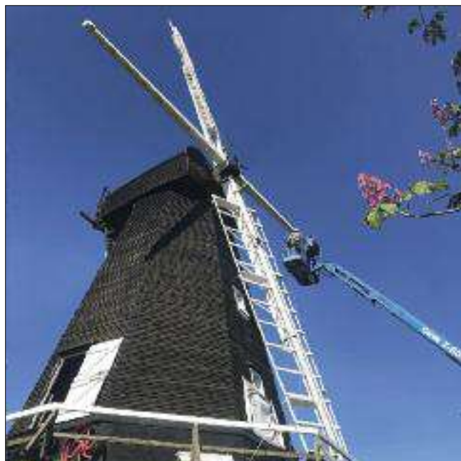
Further view of removing the sweeps from Herne Windmill. Picture – Tim Whiting.
