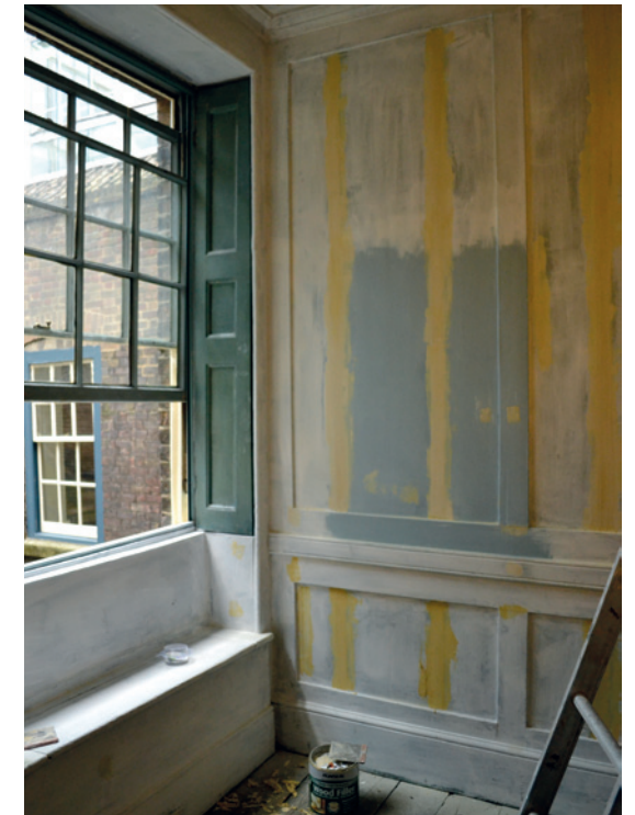
Panelling repair at No 37, prior to redecoration (SPAB).
