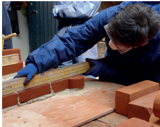
An historic brickwork masterclass at Hampton Court Palace.
