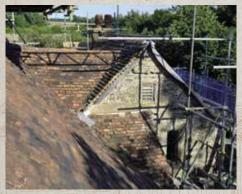
One of the building's major problems was resolved in 2020 – the repair of the roof and chimneys. New handmade tiles were fired, and lime for mortar was burnt in a kiln on site.
