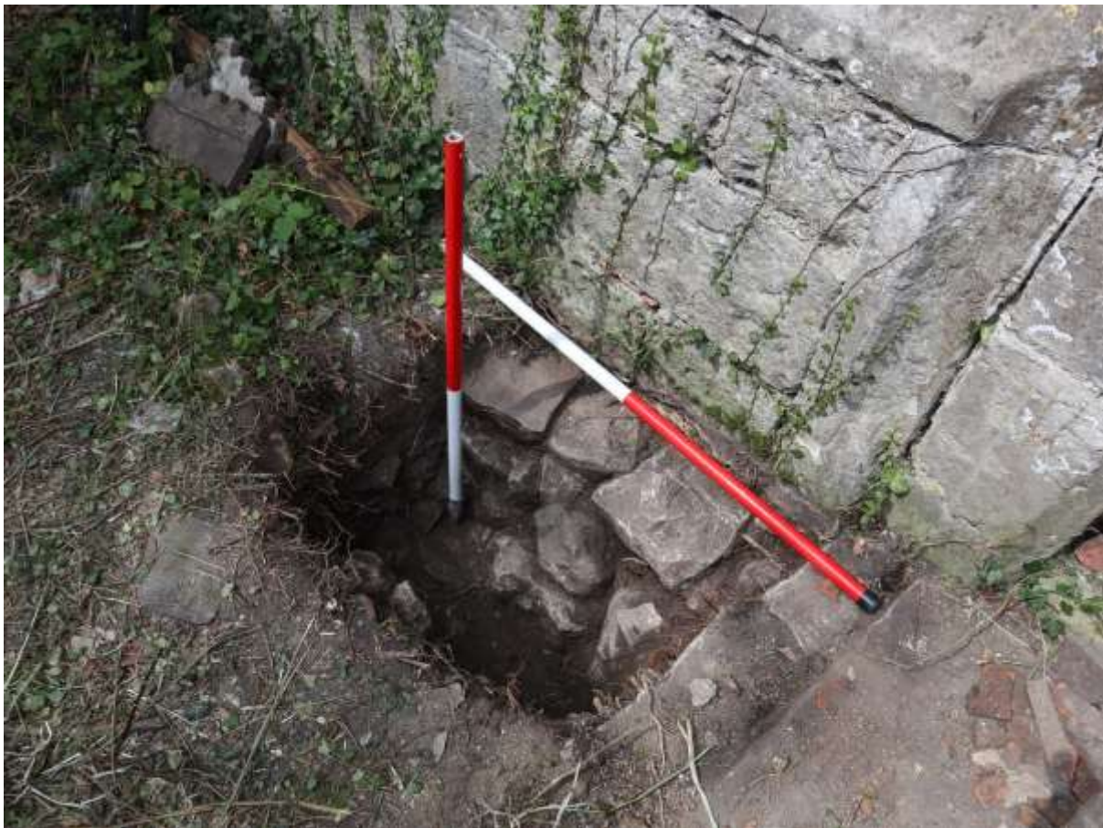
Figure 13: TP9 looking north-west, with the ragstone rubble structure (foundation?) underlying the Chapel's aisle wall, but seemingly separate from it.
