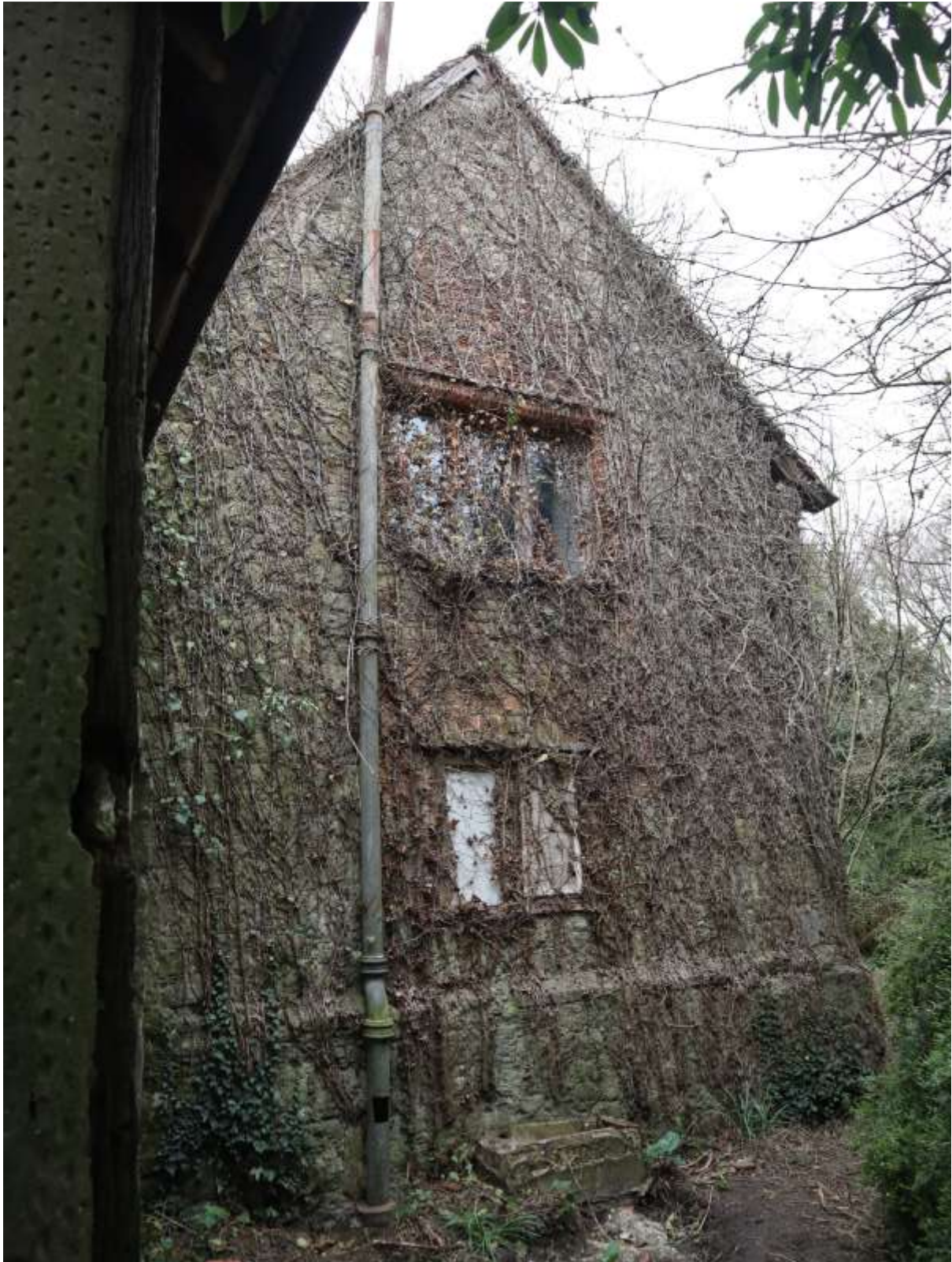
Figure 16: The east elevation of the Chapel is still obscured by ivy (now dead), but the arch of the former lancet window can still be discerned through the brick blocking above and below the first-floor window. The absence of such blocking beneath the ground-floor window suggests that its cill is at a similar (perhaps the same) height as the medieval original.
