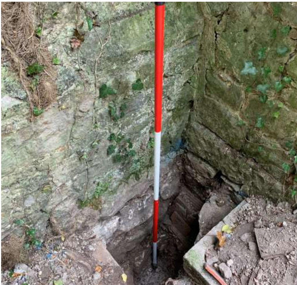
Figure 15: Evidence for what may have been an offset, now badly damaged, at or just above the current ground level can be seen in TP6. Note the way the bottom of the porch wall is 'sloped' against the wall of the Chapel. Note also the moulded chamfered plinth at a higher level in the wall behind the top of the ranging rod.
