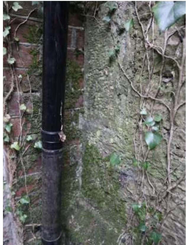
Figure 17: The relationship between the east wall of the Chapel and the brick pier at its junction with the timber framed extension to the east. The left-hand photograph shows the lower part of the pier clearly butting against the moulded plinth of the east end, but the right-hand image shows equally clearly that the fine ashlar blocks of the Chapel abut the brickwork!
