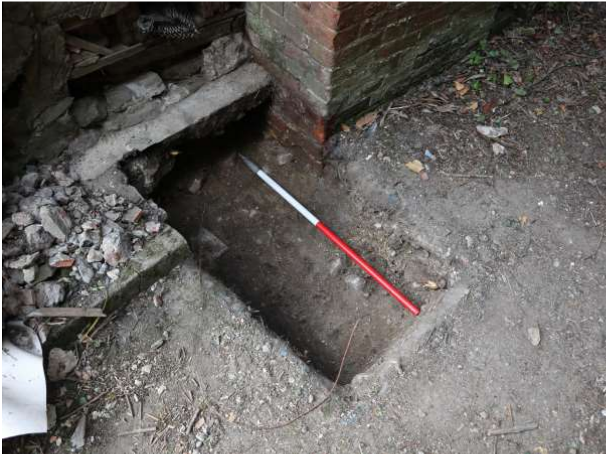
Figure 9: TP4 looking north-west, showing the bead-moulded re-used timber at the base of the framed extension, its poor-quality footings (supported by a remnant of the concrete drain), and the brick chimney stack. The layer of cobbles can just be seen under the stack.
