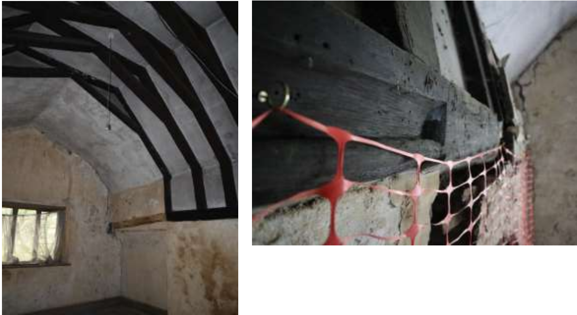
Figure 18: Left – the abrupt change from the late medieval wall and roof to the post-Dissolution west extension, evident on the north side of the Chapel. Right – the stopped moulding on the south wall plate, first floor: this would have returned across the original west end of the Chapel.
