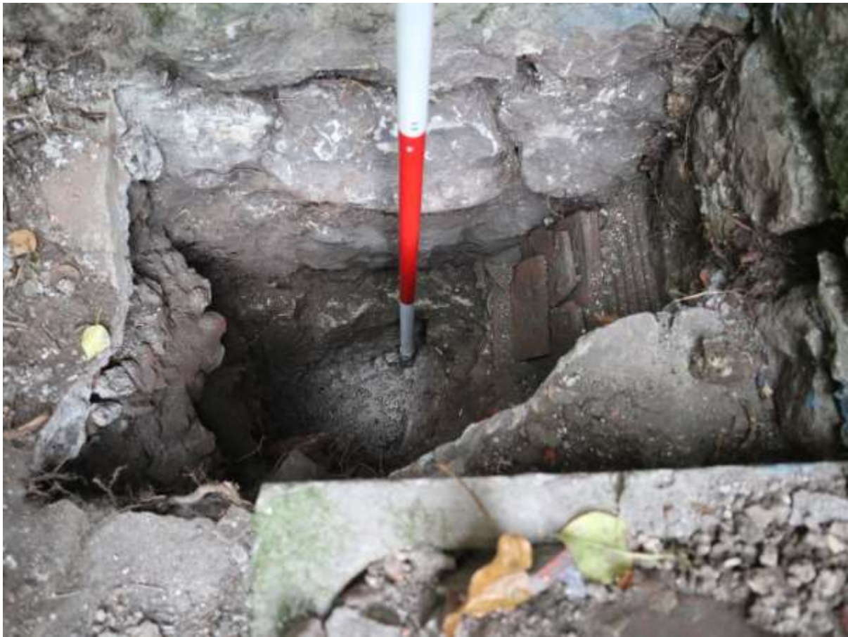
Figure 11: TP6 looking south, with the Gault Formation at the base overlain by the north wall of the Chapel. Note the stacked tile footing for the porch, overlaying the offset foundation.
