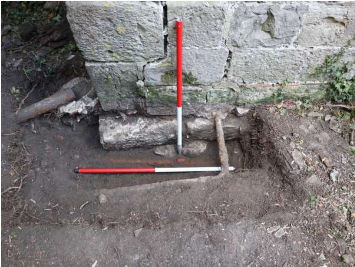
Figure 7: TP 2 looking north, with extensive movement in wall 20 and foundation 21 clearly visible. Note the isolated stones ( 22 ) under the middle of 21 , and the various modern services.
