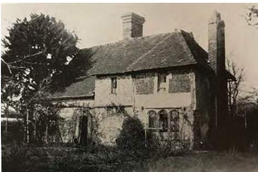
Photograph of the south elevation of St. Andrew's, c.1920. (provided by J. Garlick). Comparison with the photograph of 1911 shows that the render repair to the brickwork of the upper storey of the timber frame south east 'wing' was carried out in the second decade of the twentieth century.
