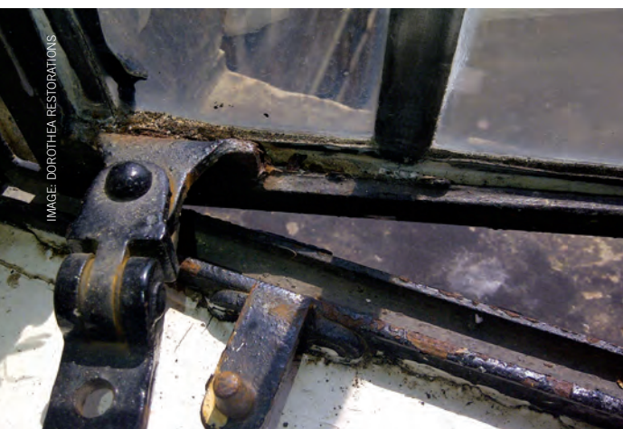
Fittings are an integral part of metal windows. Below: Early ungalvanised steel windows should be cleaned off in situ and repainted.
