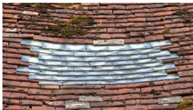
Top: This extension's casement windows reflect the proportions of the sashes in the terrace, consciously but sympathetically distinguishing new from old. Above: Glass tiles in a clay tile roof.
