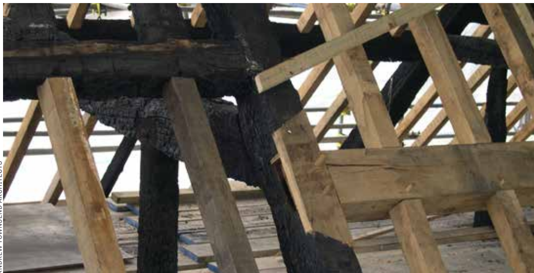
LEFT Careful roof repairs following a fire to Jordans, a Grade I listed Meeting House in Buckinghamshire.
