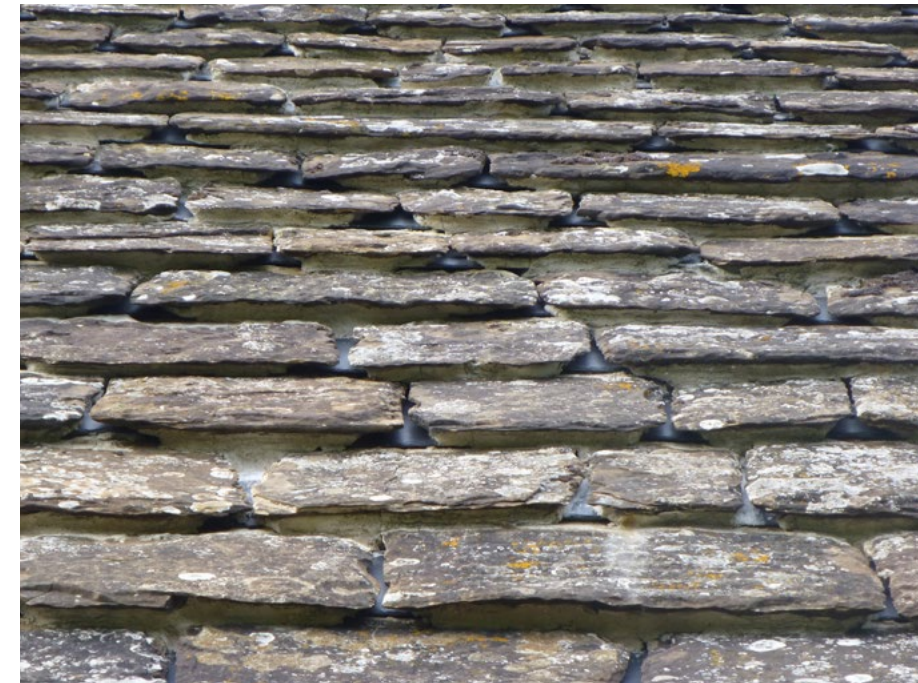
Horsham stone slate single-lapped with Welsh slate soakers at Botolphs Church, West Sussex (view angled to show technique). Photo credit: Rachel Morley.
