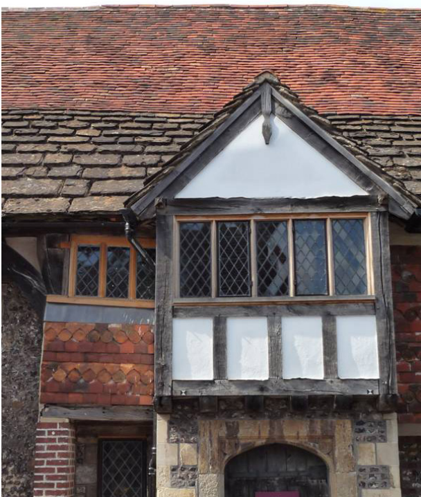
Horsham stone slate in combination with plain clay tiles at Anne of Cleves House, Lewes, East Sussex. Photo credit: Matthew Slocombe.
