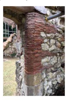
Tile repair: a method sometimes used by SPAB members to follow the eroded contours of a building and minimise fabric replacement.
