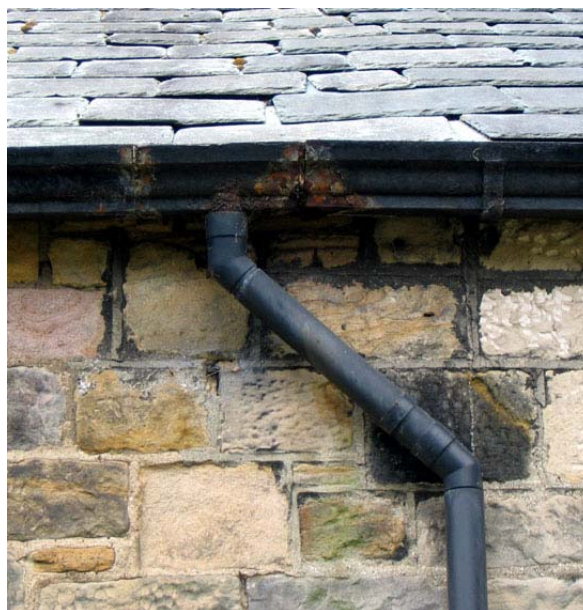
Photograph 11: Broken Gutter at Barnard Castle St Mary
