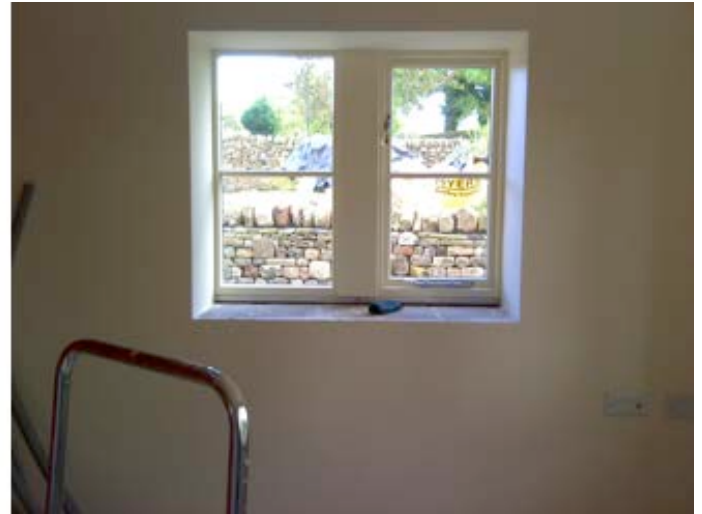
Figure 53. White House Farm, Stirton, Skipton – ingress at base of window on east wall (no sill fitted).
