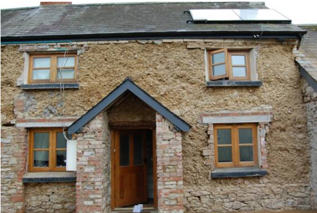
Figure 76. The Firs, Riddlecombe front elevation showing masonry buttress bottom left of frame.
