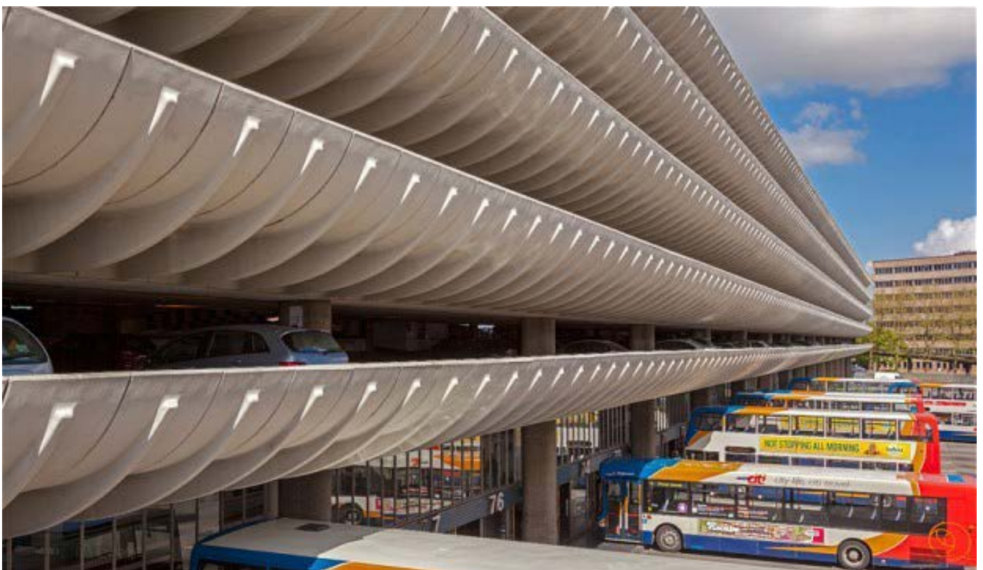
Keynote: why heritage matters Photo: Preston Bus Station – saved from demolition by a public outcry, listed at Grade II and refurbished as the result of a local and national campaign. Photo credit: The Telegraph
