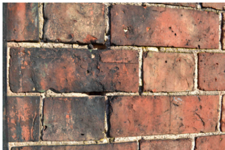
Figure 5. Bricks at Shrewsbury laid in a 'brick and a half thick' Flemish bond.
