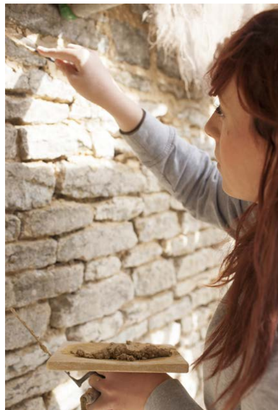
Left and right: SPAB Fellows Emily Hale repointing with lime. Photo credits: Ralph Hodgson
