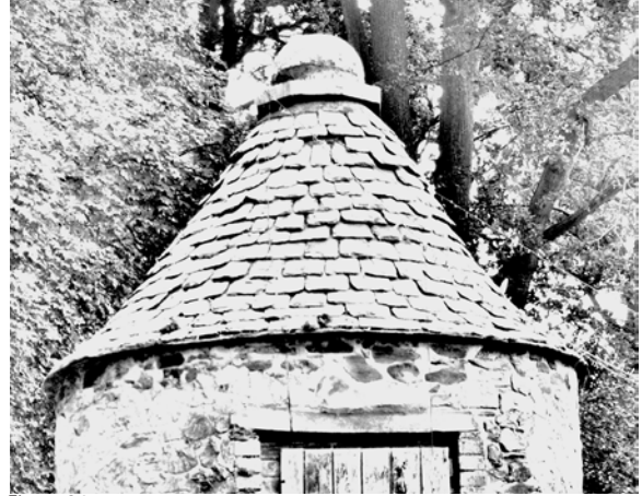
Figure 34 Curved Swithland slating is rare even though the log narrow slates are well suited to conical roofs. Terry Hughes
