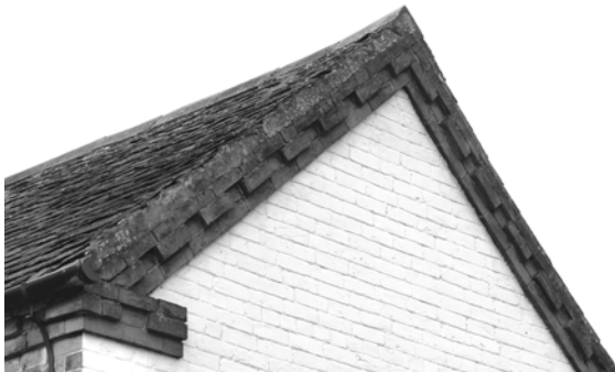
Figure 32 On later roofs verges were extended with decorative brickwork or terracotta. Terry Hughes
