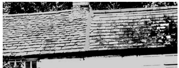
Figure 28 It is possible to obtain facsimile Swithland slates made from Welsh slate rock. However, a mix of standard sizes from the quarries stock will not produce a convincing roof. Terry Hughes
