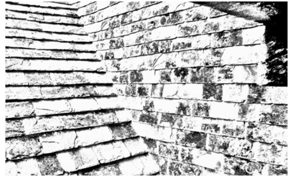
Figure 54 Wall cladding is uncommon with Collyweston slates - mainly seen on dormer cheeks. Where it is applied it is good practice to match the coursing it with the adjacent slope.
