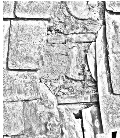
Figure 35a Mortar is used for all the normal techniques of bedding and torching. One unusual example is known, at Thorpe Satchville Church, where the slating was solid bedded in hot lime onto the ceiling laths. This was renewed as found in 2015. Terry Hughes
