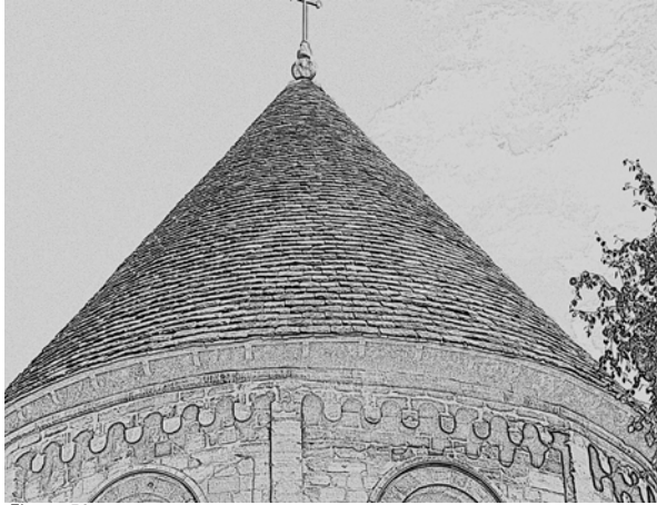
Figure 50 There are successful examples of curved Collyweston slating but they are uncommon.
