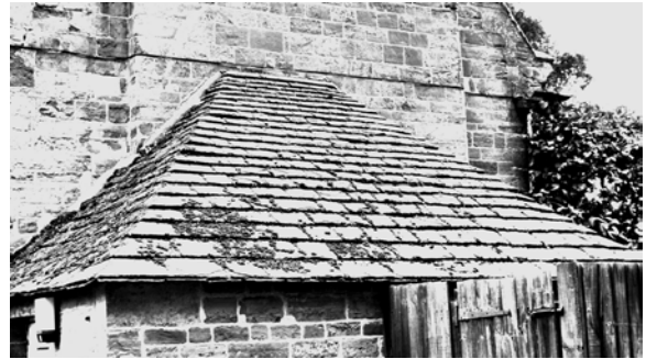
Figure 17 Mitred hips are vulnerable to wind so wide slate should be used to ensure sufficient width and therefore strength at the top of the raking cut. Terry Hughes
