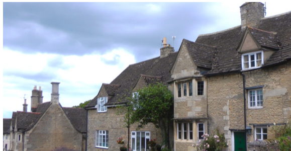
Figure 21 Collyweston dormers can be below, braking and above the eaves and monopitch, gabled or hipped.
