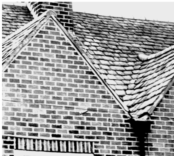
Figure 19 There are very few pre-nineteenth century Swithland roofs and those that still exist do not generally include valleys (or hips). So the valleys that are seen today - Welsh and a swept type - seem to be none-vernacular innovations. Later still even these have regrettably been replaced with open lead and close mitred types. Terry Hughes
