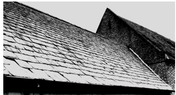
Figure 29 The eaves of swithland roofs are often formed with one or two courses of much larger and thicker slates giving the roofs a distinctive appearance. Terry Hughes
