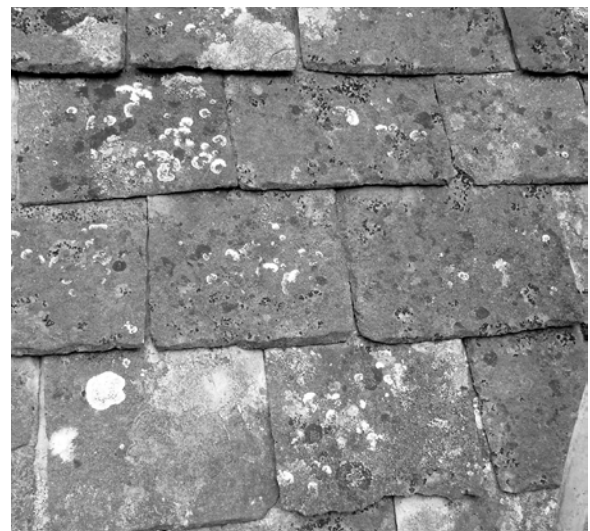
Figure 36 The texture of limestone slates varies between quite smooth, Collyweston for example, and rough for some Cotswold types and magnesian limestone. Terry Hughes
