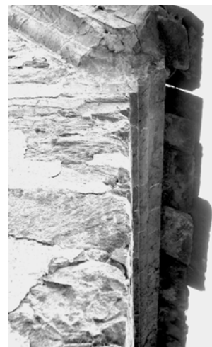
Figure 30 During the nineteenth century a large eaves overhang was formed by corbelling the wall head with decorative brickwork.
