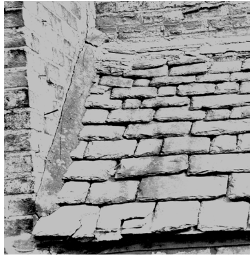
Figure 12 Before the availability or affordability of lead for soakers abutments were weathered with simple mortar flaunches. Terry Hughes
