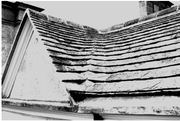
Figure 20 Collyweston slate valleys are always laced.
