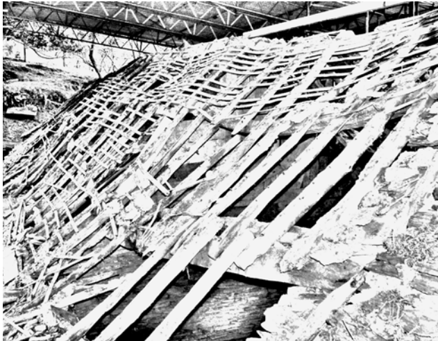
Figure 6a Movement of the roof structure may not require any correction or perhaps just stabilising. But if there are severe or abrupt undulations they can be impossible to slate over without the slates gapping even if small or narrow slates are used. In this case the undulations can be eased. Terry Hughes
