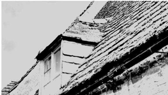
Figure 16a Where dormer ridges run into the main slating they are either swept up into the main slope or the junction is weathered with a lead saddle. Terry Hughes and Ray Harrison
