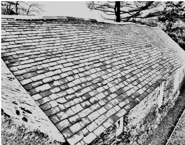
Figure 6b If undulations are only eased by the minimum to allow tight slating the roof's charm will be conserved. Terry Hughes
