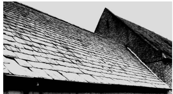
Figure 29 The eaves of swithland roofs are often formed with one or two courses of much larger and thicker slates giving the roofs a distinctive appearance.
