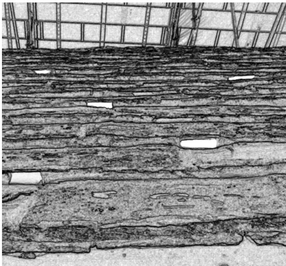
Figure 45 Fully bedded Collyweston slating is effectively sealed and cannot readily ventilate moisture from inside the roof. If ventilation is necessary small gaps can be left in the bedding. This also works as access for small bats. Terry Hughes
