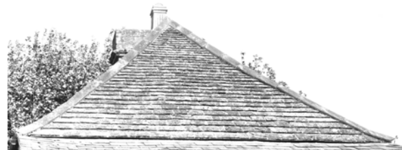
Figure 18 An alternative wind resistant hip is achieved by bedding on heavy ridge tiles supported by a hip iron at the eave. Terry Hughes
