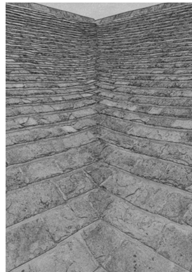
Figure 48 Collyweston valleys are always laced by laying a roughly square slates diagonally up the valley and turning the adjacent slates on each to butt up against them. Terry Hughes
