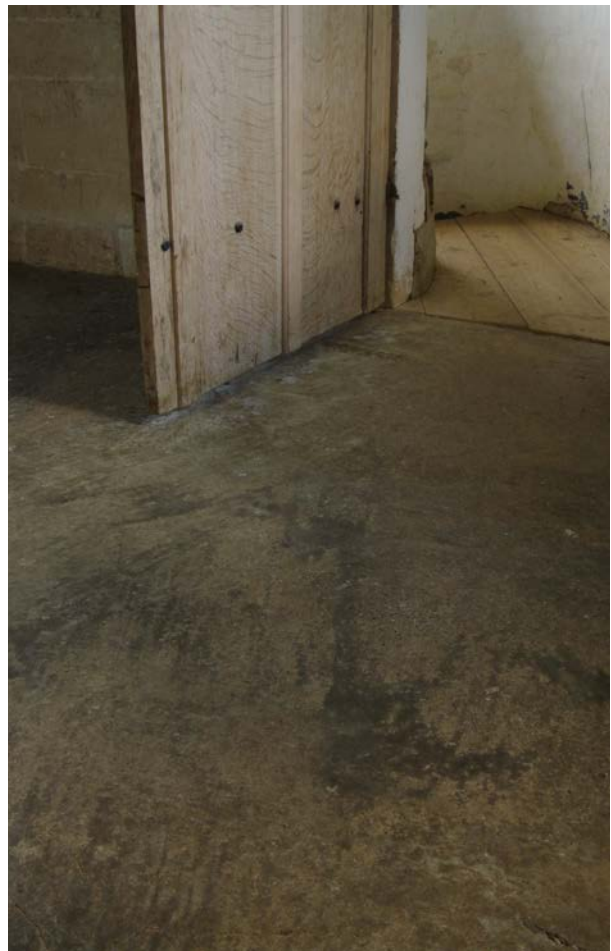
Figure 3: The patination from years of wear in a gypsum plaster floor at The Triangular Lodge in Rushton, Northamptonshire. Photo: Douglas D Kent
