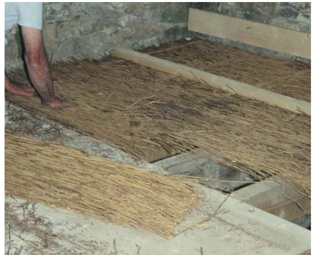
Figure 17: New reed bedding being laid.
