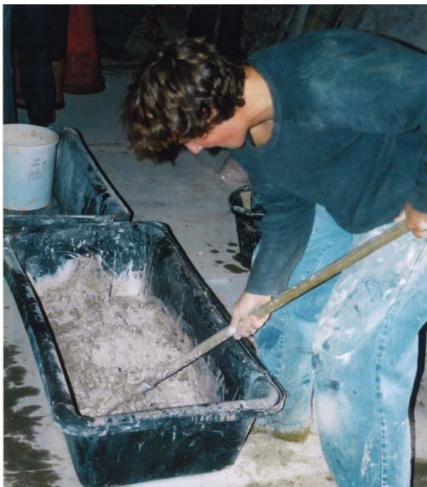
Figure 19: Mixing gypsum plaster in a plasterer's bath.
