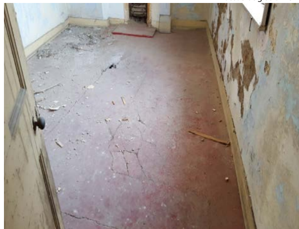
Figure 12: The nature and causes of defects should be clearly established before carrying out work involving an old gypsum plaster floor.
