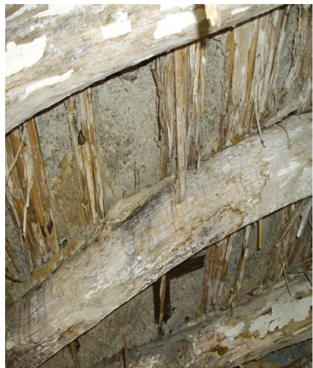
Figure 4: Cane bedding forming the underside of a historic gypsum plaster floor in Siero, Andalusia, Spain. Photo: Douglas D Kent
