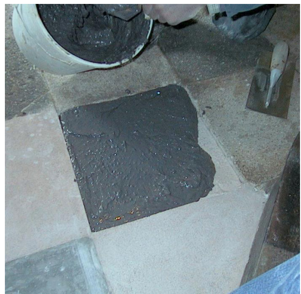
Figure 15: Materials and methods for repairs should match those of the original gypsum plaster floor as far as possible. Photo: A J Goode Ltd
