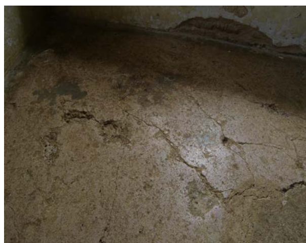
Figure 11: An old gypsum plaster floor may look beyond repair but can frequently be brought back into a sound, functioning condition.
