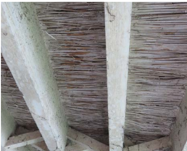
Figure 2: The presence of organic bedding material, such as reed, can indicate the existence of a gypsum plaster floor. Photo: A J Goode Ltd
