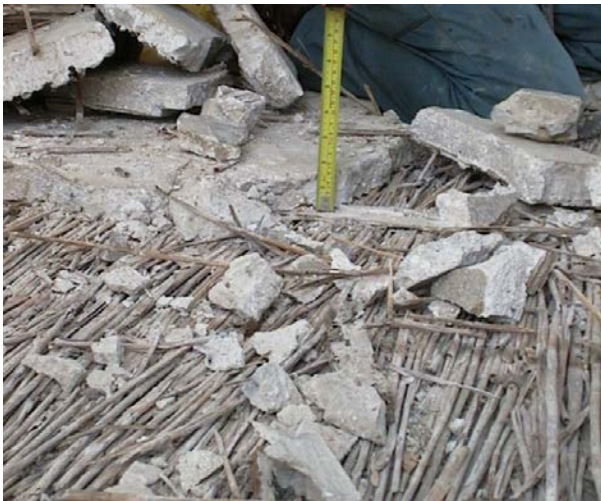
Figure 16: Old gypsum plaster that is removed should normally be retained for use as aggregate when laying replacement flooring. Photo A J Goode Ltd
