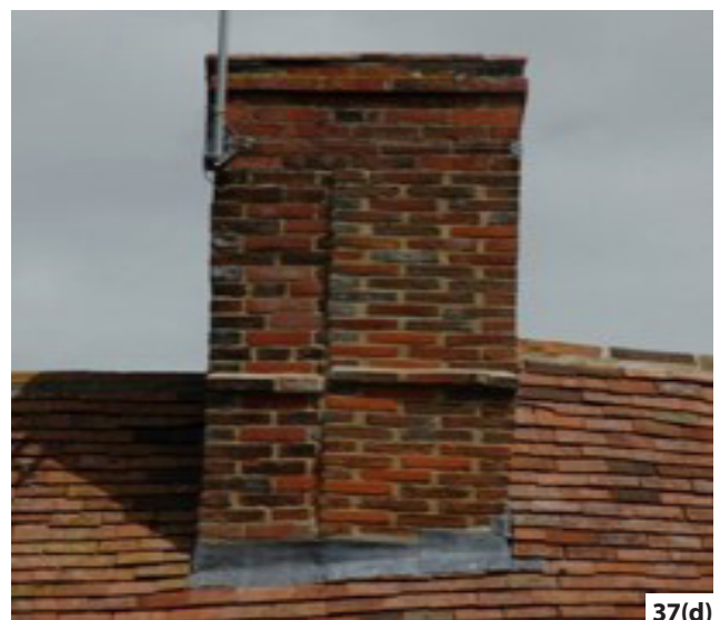
Figure 37: Chimney termination: (a) The stack shown in figure 34 from above. Note the exposure to the weather and previous attempts at repair using cement-based mortars. (b) The top of the stack protected with new stone slabs. The two redundant flues have complete slabs, the working flue has a stone capping to the brickwork. (c) The redundant flues have air slots to prevent condensation. (d) The finished stack, repaired using hydraulic lime mortar.
