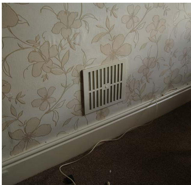
Figure 38: A redundant flue should be ventilated at the bottom where the fireplace opening is blocked off.
