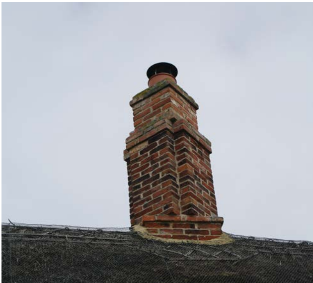
Figure 31: Chimney height raised on thatched cottage.
