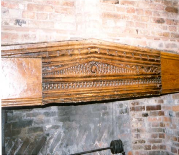
Figure 17: Repair is preferable to replacement, as with the repaired ends of this mantel beam. They respect the original but do not attempt to ape it. Photo: © Douglas D Kent
