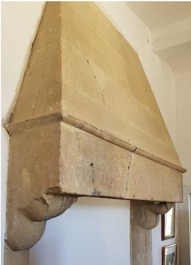
Figure 3: Corbelled stone hood, c1315. Gatehouse, Ham Court, Bampton, Oxfordshire.
