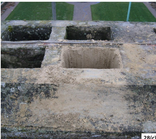
Figure 28: Re-parging of flue: (a) Winch for drawing up sponge. (b) New parging mortar applied. (c) Only one flue remains in use, the other flues have not been relined.
