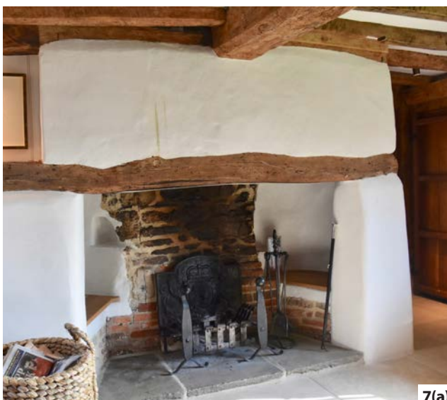
Figure 7: Inglenook fireplaces: (a) South Oxfordshire, c1600s, with seat alcoves either side for enjoying the warmth of the fire. The original flagstones under the grate would have been flush with the floor to allow debris to be swept into the hearth. (b) Kitchen fireplace, c1550, with pot crane, bread oven and cast iron fireback. Pendean, Weald and Downland Living Museum, West Sussex. Photos: Marianne Suhr (a) and Sally Stradling, with thanks to Weald and Downland Living Museum (b)
