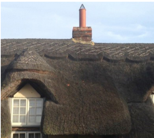
Figure 32: A chimney terminating less than the recommended 1.8 m above the ridge of a thatched building. The top of the terminal with an uninsulated pot is taken as being 150 mm above its base. The addition of a bird guard will reduce fire risk.
