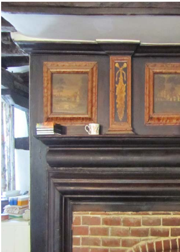
Figure 10: Detail, fireplace with bolection moulding, c1700s. Stevenston, Oxfordshire. Photo: Sally Stradling
