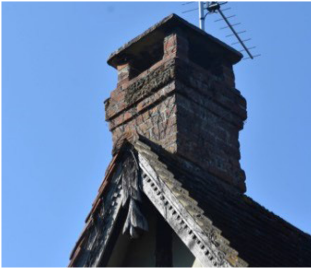
Figure 21: A 'dovecote' top can be used to protect large flue outlets from wind and rain, though is inadvisable on thatched buildings. A stone slab is placed above the flue opening raised on bricks at the corners. Such terminations should incorporate suitable bird mesh to stop nests being built under the slab. However, addition of a slab roof may affect the draw in certain situations. Always light a fire and check for unintended consequences before striking the scaffolding around the stack.
