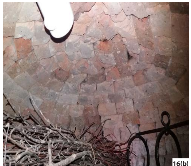
Figure 16: Bread ovens: (a) Bread oven 'bulge'. East Hanney, Oxfordshire. (b) Interior of bread oven showing brick lining. Old Priest's House, West Hoathly, West Sussex
