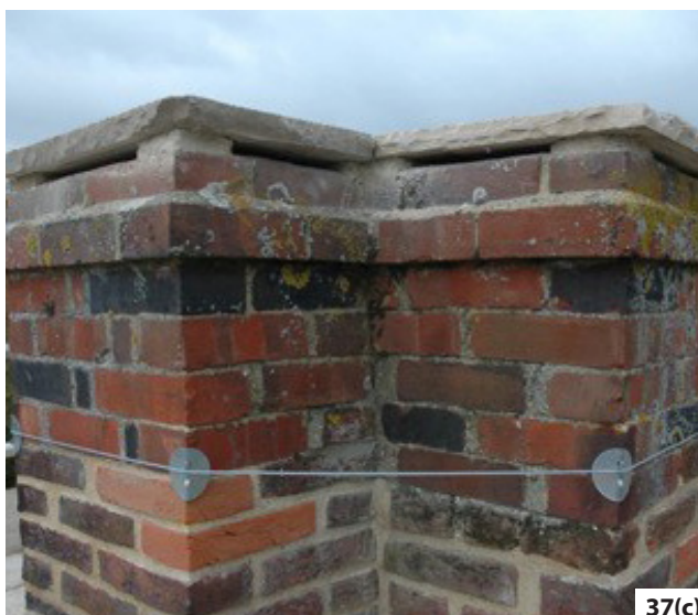
Figure 37: Chimney termination: (a) The stack shown in figure 34 from above. Note the exposure to the weather and previous attempts at repair using cement-based mortars. (b) The top of the stack protected with new stone slabs. The two redundant flues have complete slabs, the working flue has a stone capping to the brickwork. (c) The redundant flues have air slots to prevent condensation. (d) The finished stack, repaired using hydraulic lime mortar.
