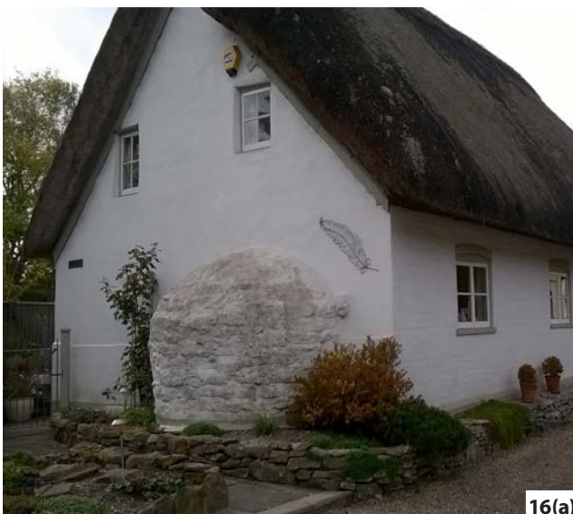
Figure 16: Bread ovens: (a) Bread oven 'bulge'. East Hanney, Oxfordshire. (b) Interior of bread oven showing brick lining. Old Priest's House, West Hoathly, West Sussex
