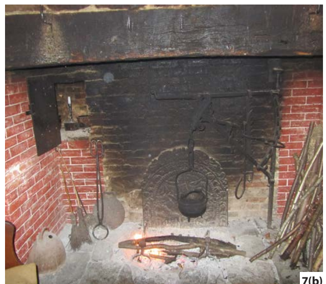
Figure 7: Inglenook fireplaces: (a) South Oxfordshire, c1600s, with seat alcoves either side for enjoying the warmth of the fire. The original flagstones under the grate would have been flush with the floor to allow debris to be swept into the hearth. (b) Kitchen fireplace, c1550, with pot crane, bread oven and cast iron fireback. Pendean, Weald and Downland Living Museum, West Sussex. Photos: Marianne Suhr (a) and Sally Stradling, with thanks to Weald and Downland Living Museum (b)
