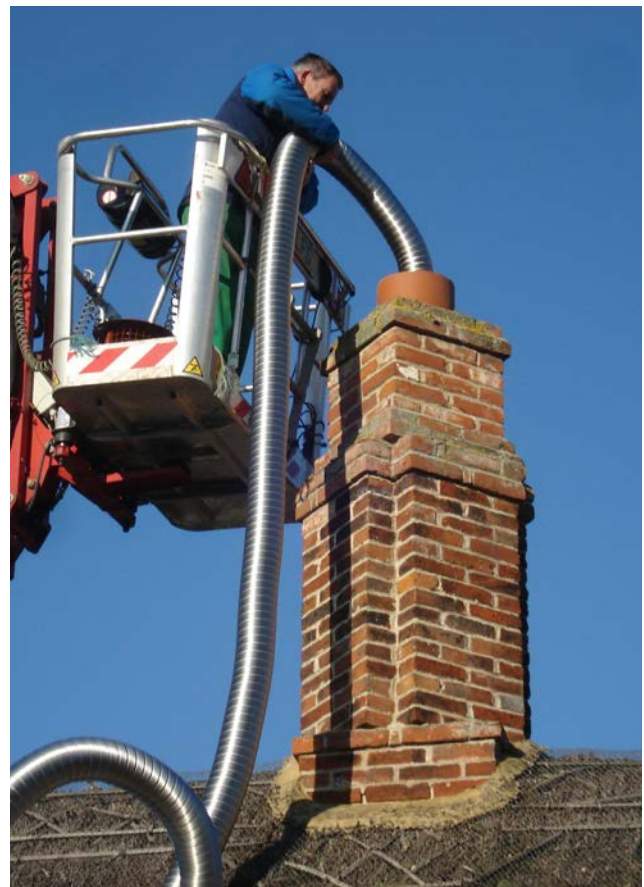
Figure 29: Flexible metal liner being inserted into chimney of thatched cottage to serve new gas stove after removal of a wood burner to reduce the fire risk.
