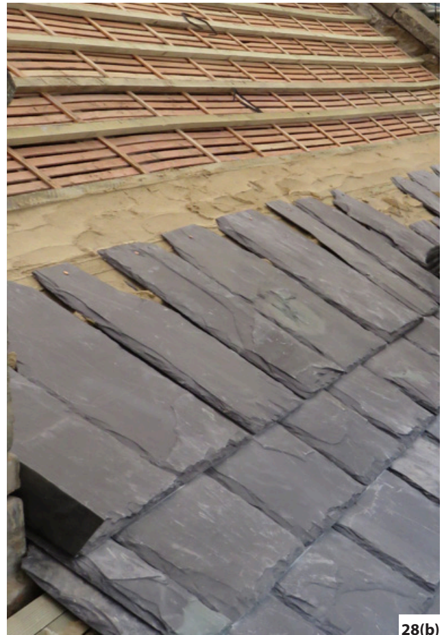
Figure 28: Mortar is used for all the normal techniques of bedding and torching. One unusual example is known, at St Michael and All Angels' Church in Thorpe Sackville, Leicestershire. The slating was solid-bedded in hot lime onto the ceiling laths (a). This was renewed as found (b). Photos: Terry Hughes
