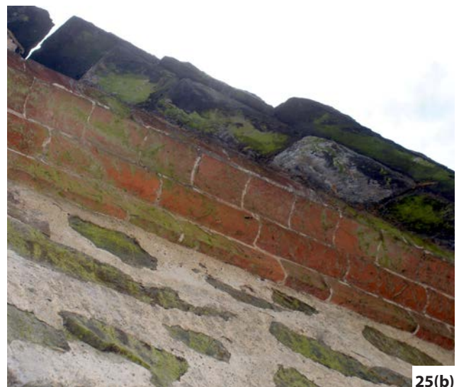
Figure 25: The eaves of Swithland roofs are often formed with one or two courses of much larger and thicker slates, giving the roofs a distinctive appearance (a). During the 19th century, a large eaves overhang was formed by corbelling the wallhead with decorative brickwork (b). Photos: Terry Hughes
