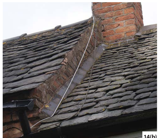
Figure 14: Abutments: (a) Before the availability or affordability of lead for soakers, abutments were weathered with simple mortar fillets. (b) Because fillets are prone to cracking and leaks, one technique to help prevent this is to bed slates, thin stones or tiles into the mortar. In some regions these are known as listings.
