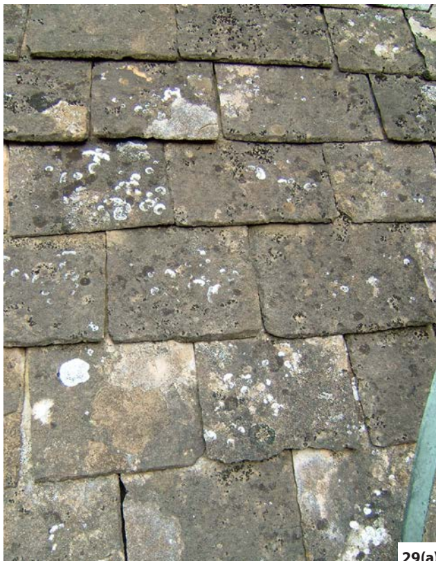
Figure 29: The texture of limestone slates varies between quite smooth (a), to rough, as with some Cotswold types and Magnesian limestone (b)
