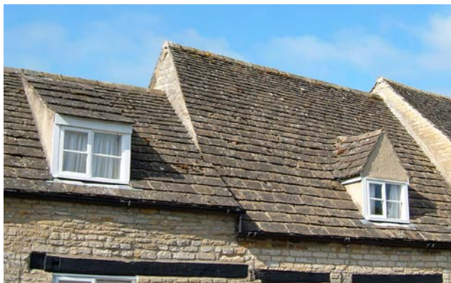
Figure 37: Dormer windows are common in Collyweston roofs and the full range of types – monopitched, gabled and hipped – are commonly positioned below, breaking and above the eaves and in the roof slope. Photo: Terry Hughes
