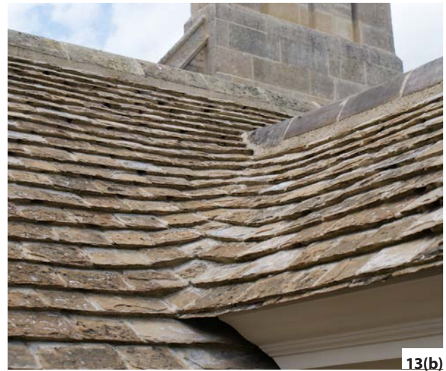
Figure 13: Valleys: (a) There are very few pre-19th-century Swithland roofs and those that still exist do not generally include valleys (or hips). The valleys that are seen today – Welsh and a swept type – seem to be non-vernacular innovations. Later still, even these have regrettably been replaced with open lead and close-mitred types. (b) Collyweston Slate valleys are always laced.
