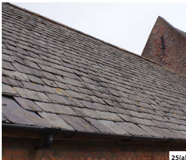
Figure 25: The eaves of Swithland roofs are often formed with one or two courses of much larger and thicker slates, giving the roofs a distinctive appearance (a). During the 19th century, a large eaves overhang was formed by corbelling the wallhead with decorative brickwork (b). Photos: Terry Hughes
