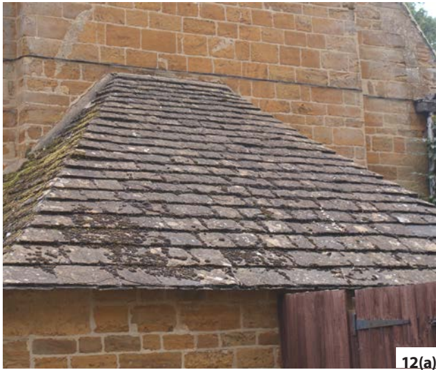
Figure 12: Hips: (a) Mitred hips are vulnerable to wind so wide slates should be used to ensure sufficient width and, therefore, strength, at the top of the raking cut. (b) An alternative wind-resistant hip is achieved by bedding on heavy ridge tiles supported by a hip iron at the eaves.
