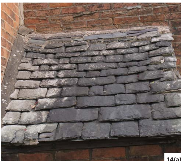
Figure 14: Abutments: (a) Before the availability or affordability of lead for soakers, abutments were weathered with simple mortar fillets. (b) Because fillets are prone to cracking and leaks, one technique to help prevent this is to bed slates, thin stones or tiles into the mortar. In some regions these are known as listings.
