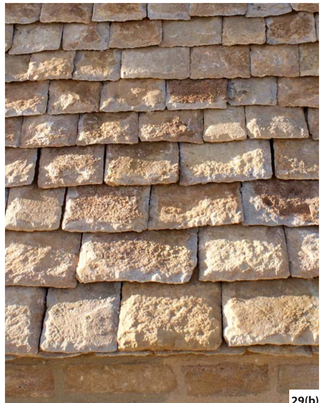
Figure 29: The texture of limestone slates varies between quite smooth (a), to rough, as with some Cotswold types and Magnesian limestone (b)
