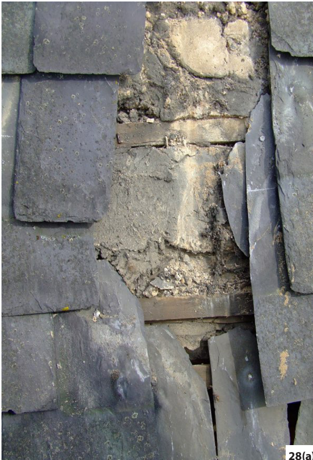
Figure 28: Mortar is used for all the normal techniques of bedding and torching. One unusual example is known, at St Michael and All Angels' Church in Thorpe Sackville, Leicestershire. The slating was solid-bedded in hot lime onto the ceiling laths (a). This was renewed as found (b). Photos: Terry Hughes
