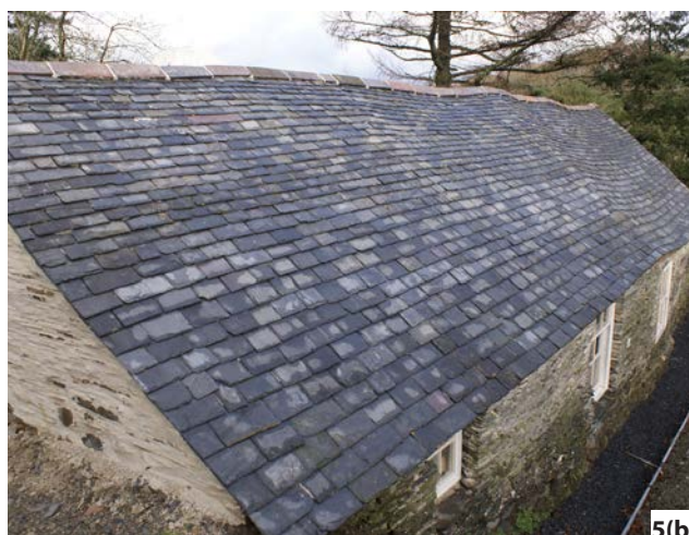
Figure 5: Movement of the roof structure: (a) Distortion may not require any correction or perhaps just needs stabilising. If there are severe or abrupt undulations, though, they can be impossible to slate over without the slates gapping, even if small or narrow slates are used. In this case the undulations can be eased. (b) If undulations are eased only by the minimum necessary to allow tight slating, the special interest of the roof will be conserved.
