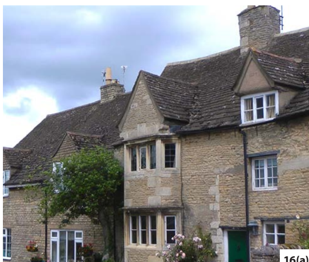
Figure 16: Dormers: (a) Collyweston dormers can be below, breaking or above the eaves and are monopitch, gabled or hipped. (b) Dormer ridges were traditionally swept up into the main roof slope. Photos: Terry Hughes
