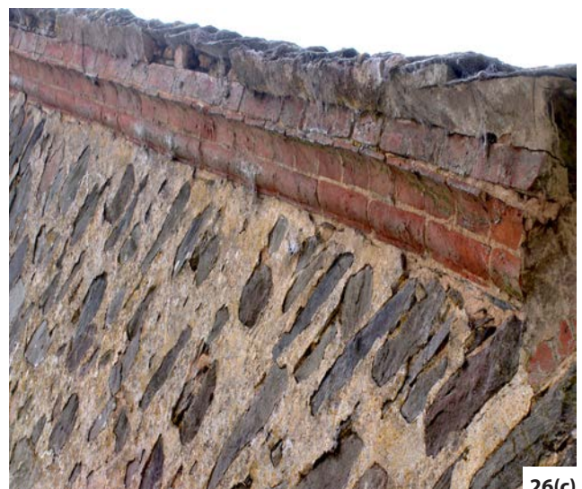
Figure 26: On early roofs, verges simply oversailed the wall by a few inches (75 mm or so) with a mortar fillet under the slate (a). With later roofs, verges were extended with decorative brickwork or terracotta (b and c).
