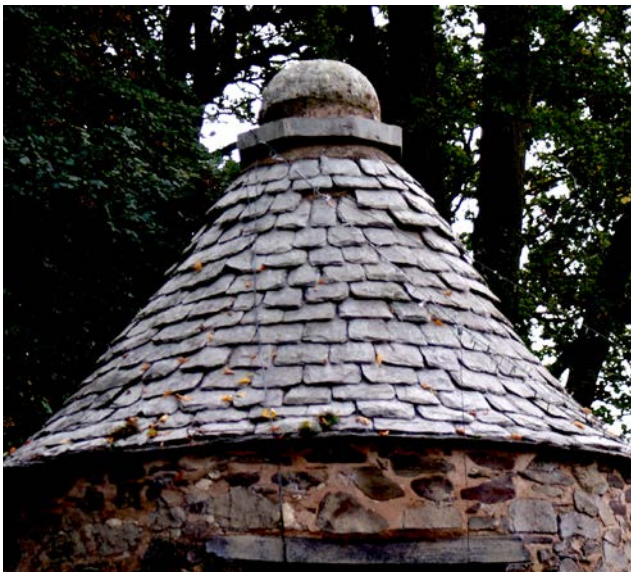
Figure 27: Curved Swithland slating is rare even though the long narrow slates are well-suited to conical roofs. Photo: Terry Hughes
