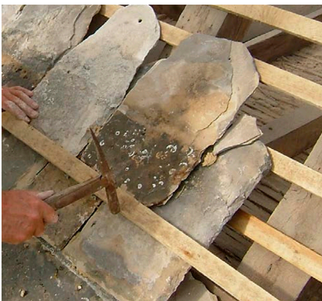
Figure 33: Shales or shadows are bedded in a small amount of mortar as the slates are laid to support their span from tail to bed. Photo: Terry Hughes
