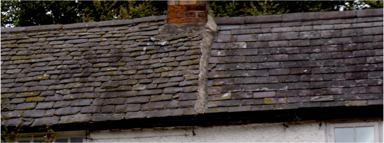
Figure 24: It is possible to obtain facsimile Swithland Slates made from Welsh slate rock. However, a mix of standard sizes from the stock at a quarry will not produce a convincing roof. Photo: Terry Hughes
