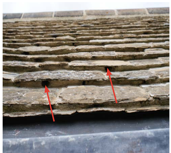
Figure 32: Fully bedded Collyweston slating is effectively sealed and cannot readily ventilate moisture from inside the roof. If ventilation is necessary, small gaps (see arrows) can be left in the bedding. This also works as access for small bats. Photo: Terry Hughes
