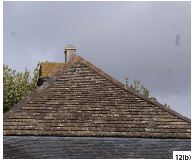
Figure 12: Hips: (a) Mitred hips are vulnerable to wind so wide slates should be used to ensure sufficient width and, therefore, strength, at the top of the raking cut. (b) An alternative wind-resistant hip is achieved by bedding on heavy ridge tiles supported by a hip iron at the eaves.
