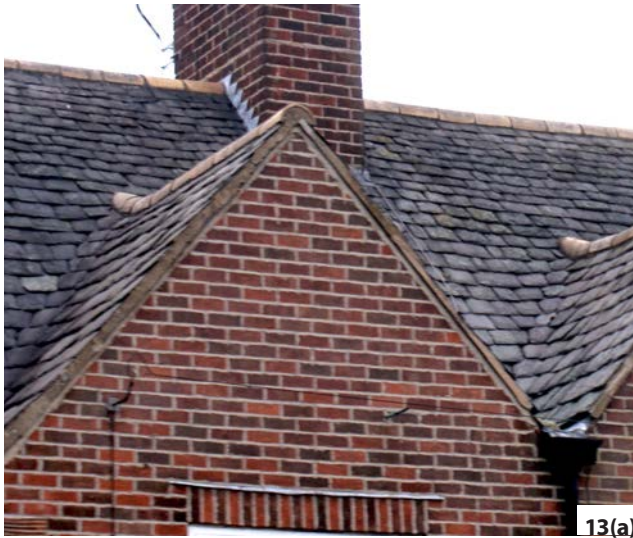
Figure 13: Valleys: (a) There are very few pre-19th-century Swithland roofs and those that still exist do not generally include valleys (or hips). The valleys that are seen today – Welsh and a swept type – seem to be non-vernacular innovations. Later still, even these have regrettably been replaced with open lead and close-mitred types. (b) Collyweston Slate valleys are always laced.
