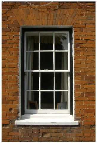
Figure 19: Windows post-dating the 18th century arecommonly made of softwood and require regular redecorationfor protection.Photo: Douglas Kent
