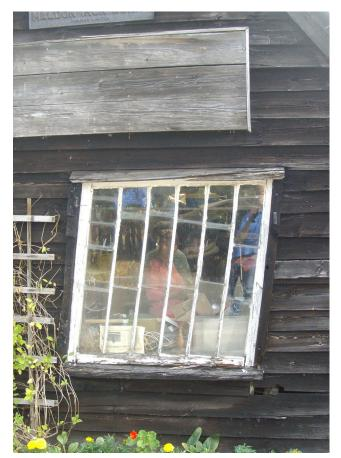
Figure 6: Structural movement.
