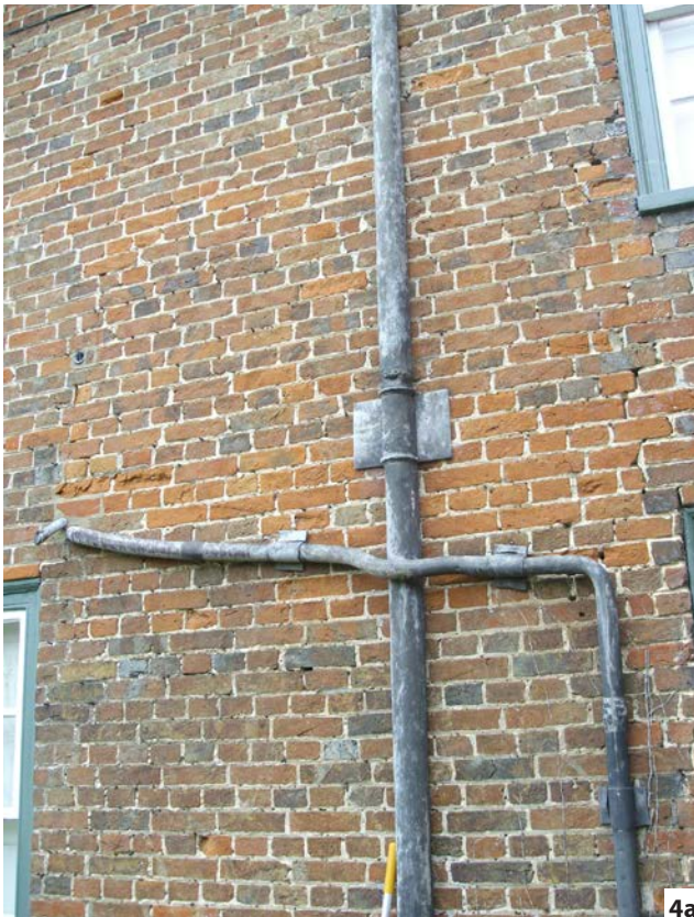
Figure 4: Lead drainage pipes: (a) Rainwater and waste water disposal. (b) For air venting, incorporating roof flashing.
