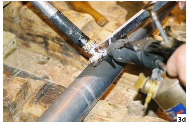
Figure 3: Formation of a branch wiped joint demonstrated on an SPAB course: (a) Opening up to receive the branch pipe. (b) Use of compasses and a scribing plate to incise the line of the joint. (c) Scraping back the masking fluid. (d) Applying the solder. Photos: Douglas D Kent
