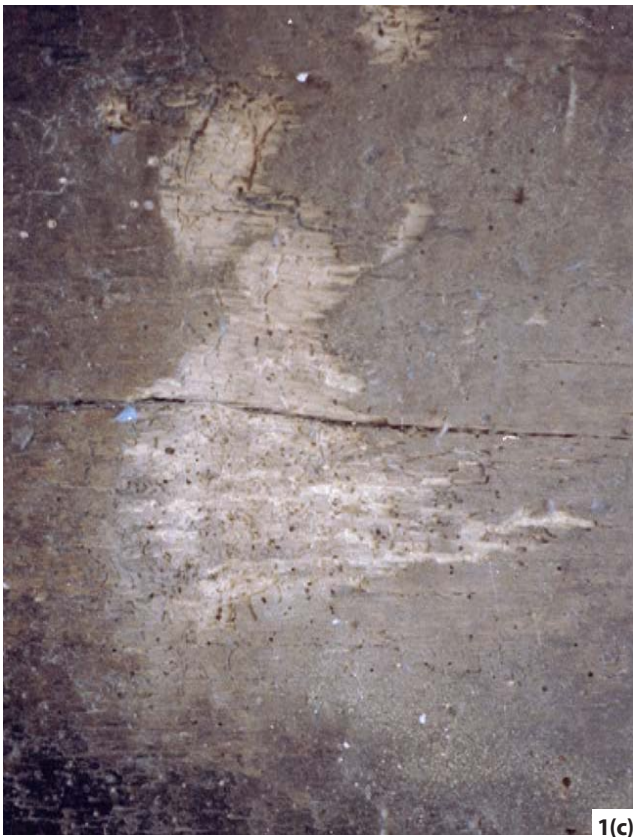
Figure 1: Damage to boards caused by: (a) and (b) Careless lifting and relaying during installation of central heating and wiring runs. (c) A castor, which can be particularly serious when the castor is positioned over the edge of a board. Softwood boards have been used inappropriately in (d) to replace a damaged wide elm board – could it have not been repaired? Photos: Philip Hughes
