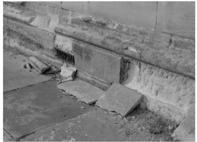
Figure 11: Salt crystallisation behind the strong cement patches on this plinth has led to both these being forced off and to further disintegration of the stonework. Photo: Philip Hughes
