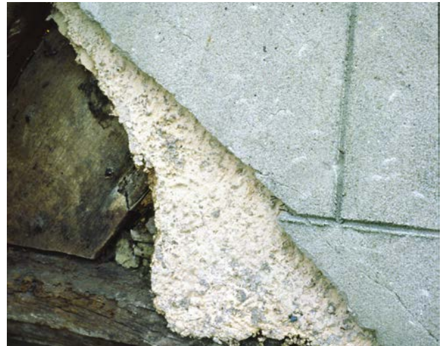
Figure 13: Cement render has been applied over a lime roughcast on this timber-framed building. The cement is being carefully removed in small pieces by forming hairline cracks with a lump hammer. Photo: Philip Hughes
