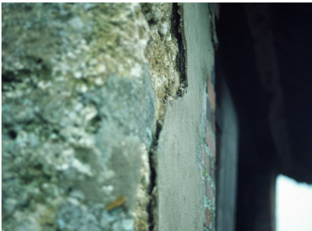
Figure 5: Strong cement render on a cob wall. The render is being forced off the wall and is taking the surface of the cob with it. The cob behind this is decaying. Photo: Philip Hughes
