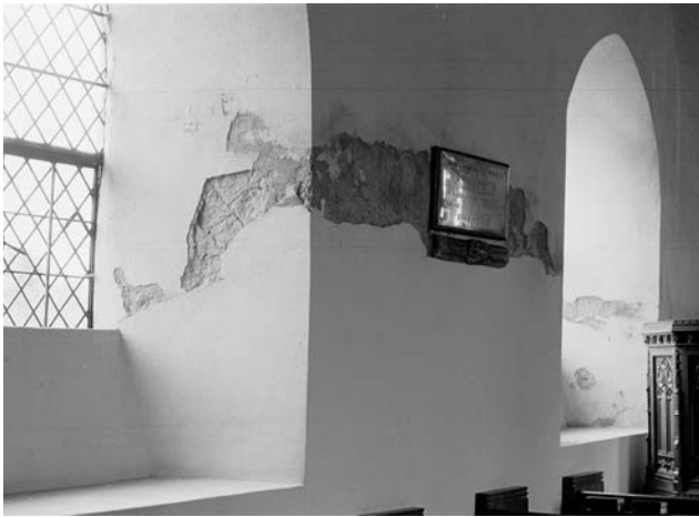
Figure 10: Strong cement-based render has been used to replace plaster affected by dampness on the lower part of these massive walls. As a result the dampness has risen higher in the wall and has now affected the old plaster that had remained sound. Photo: Philip Hughes
