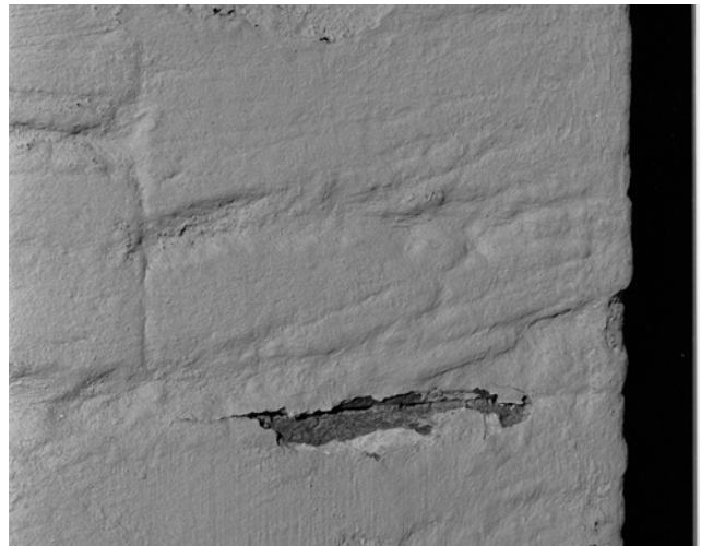
Figure 4: Moisture trapped behind an impervious paint film has caused it to blister. The effect of salts and frost has led to further decay. Photo: Philip Hughes
