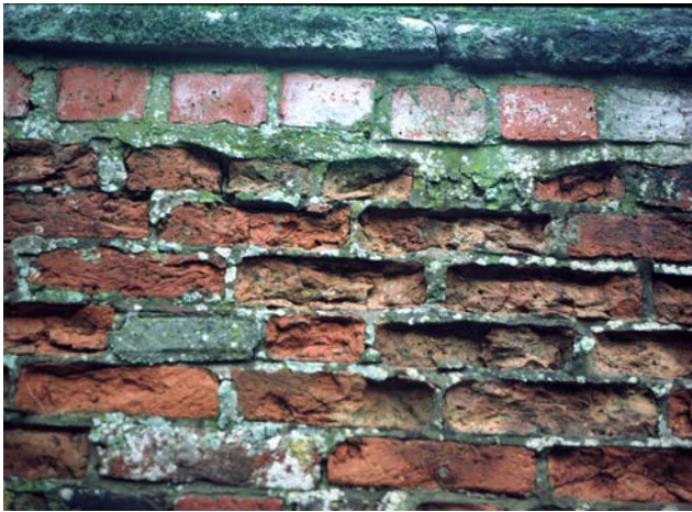
Figure 7: Strong cement-based mortar survives while the wall it was used to point up decays. This could have been avoided by the use of a lime-based mortar, weaker than the brickwork. Photo: Philip Hughes
