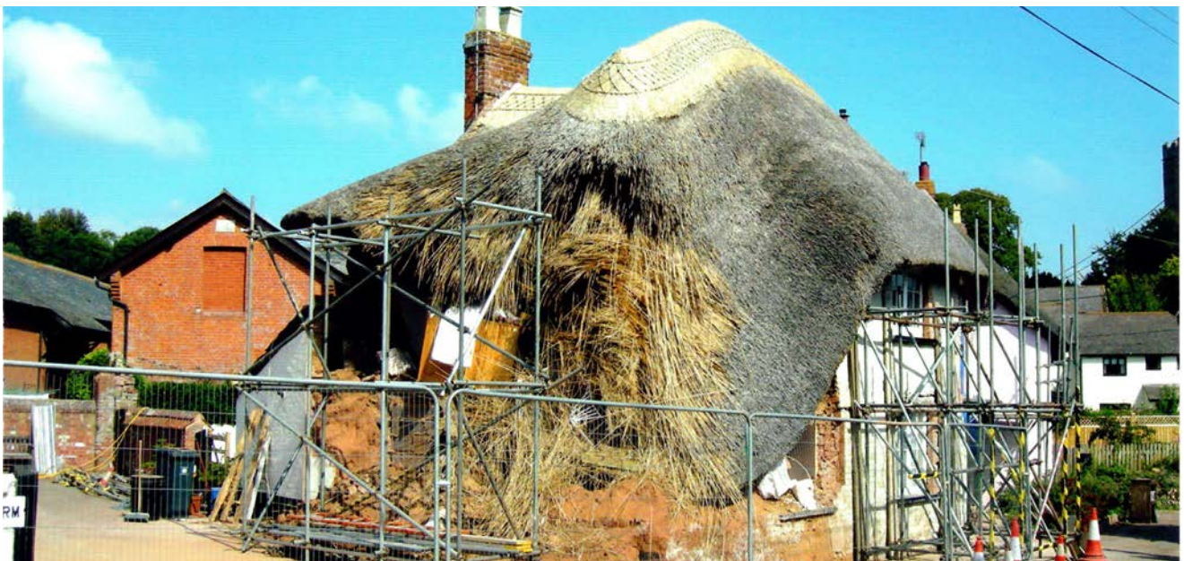
Figure 2: Water penetration has resulted in the decay of these cob walls. The cement render applied externally prevented them from drying out and led to the suddenness of the collapse. Photo: Chris Shapland
