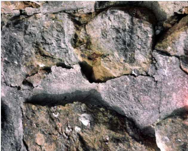
Figure 12: Strong cement pointing being forced off the wall by crystallisation of salts behind. Increased levels of dampness within the wall have caused decay of the earth-lime mortar, leading to compaction of the wall – also forcing off the dense cement pointing. Photo: Philip Hughes
