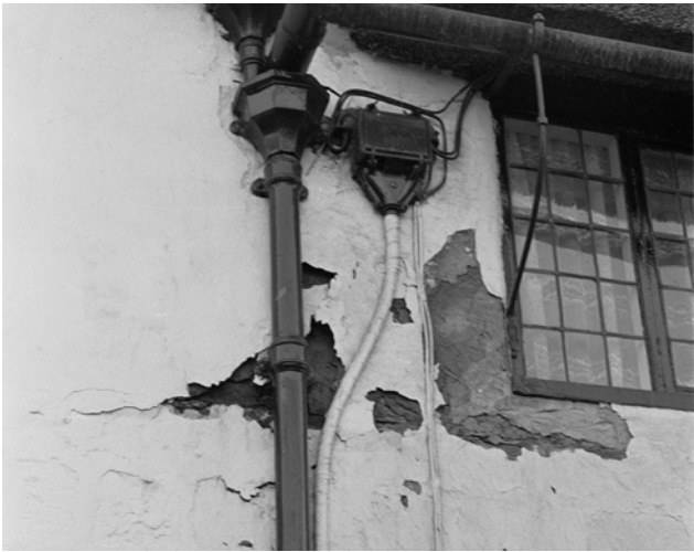
Figure 3: Frequently overflowing hopper head and gutter have saturated the wall behind an impervious paint layer. Decay of the walling immediately behind the paint film has resulted in flaking. Photo: Philip Hughes
