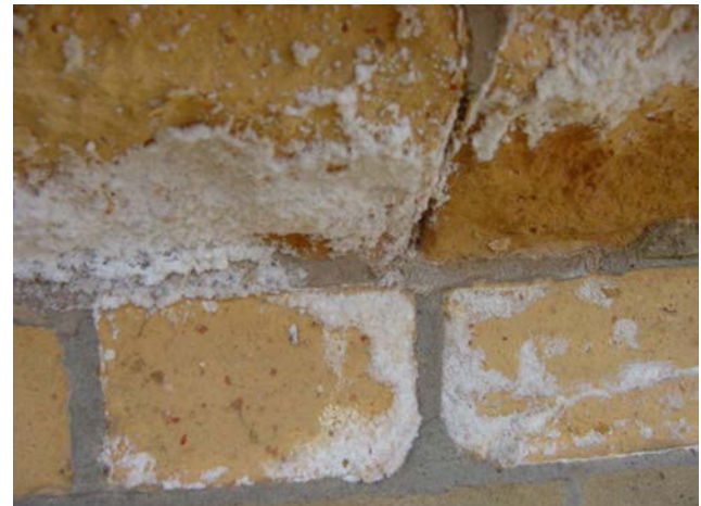
Figure 8: This wall has been repointed in a cement-based mortar. It is suffering severely from the deposition of salts. Efflorescence is occurring on the surface of the bricks instead of on the mortar joints as would be the case had a porous lime mortar been used. Photo: Philip Hughes
