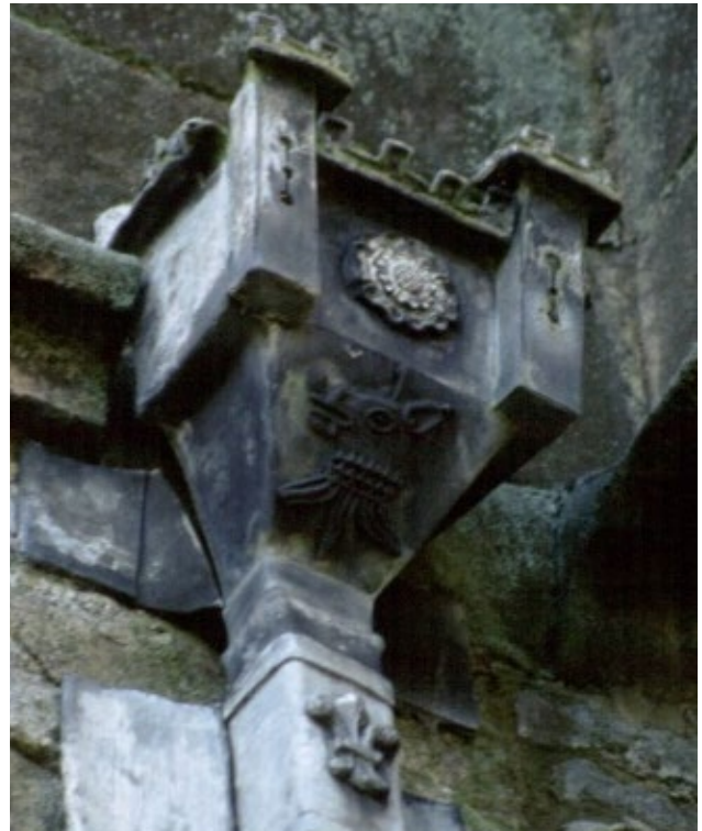
Figure 7: Sixteenth-century rainwater head showing two castellated bartizans, cast Tudor rose and fleur-de-lis, Haddon Hall, Derbyshire. Photo: Peter T J Rumley
