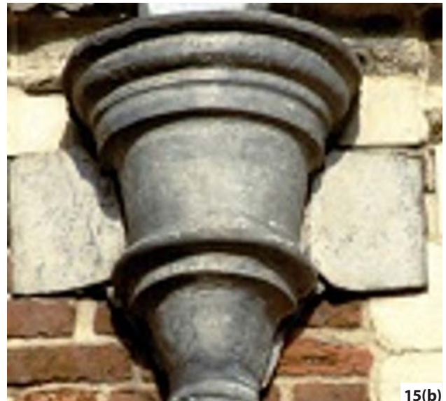
Figure 15: Formation of a decorative rainwater head: (a) Half-round wooden block over which lead is dressed. (b) Half-round 18th-century rainwater head having been dressed over wooden block at 16 Watling Street, Canterbury, Kent. Photos: Peter T J Rumley
