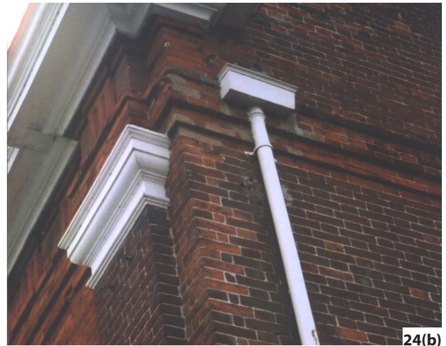
Figure 24: Avoidable loss of a rainwater head: (a) Eighteenth-century original. (b) Inappropriate replacement.
