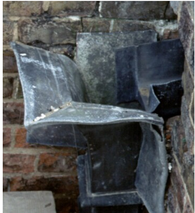
Figure 23: Torn lead cornice of rainwater head, prior to repair. Tilbury Fort, Essex. Photo: Peter T J Rumley
