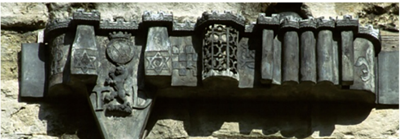
Figure 8: Tinning of stars, chequerwork, strapwork and, far right, fleur-de-lis on a rainwater head that incorporates eight battlemented bartizans, the third from the right pierced. The date, initials, crest and leopard rampant are cast and soldered. Stone Court, Knole, Kent, 1605. Photo: Peter T J Rumley
