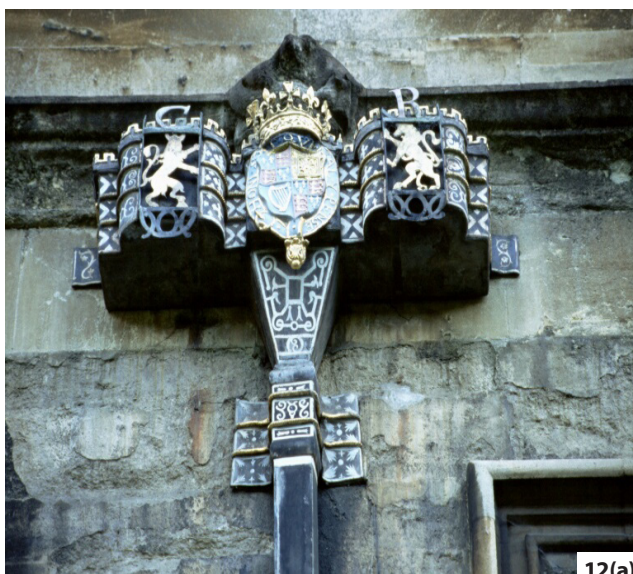
Figure 12: Rainwater heads at St John's College, Oxford, 1635: (a) With gilded unicorn cut from sheet lead and set in front to provide depth and shadows. (b) Gilded and painted. Photos: Peter T J Rumley
