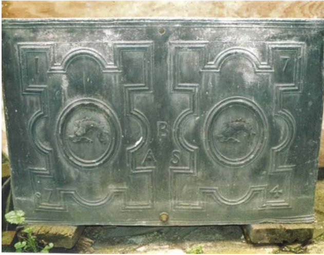
Figure 6: Sand-cast lead cistern of 1774 embellished with strapwork and motifs. Photo: Douglas D Kent
