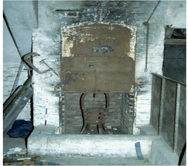
Figure 14: Nineteenth-century lead furnace (disused) at Exeter Cathedral. Photo: Peter T J Rumley
