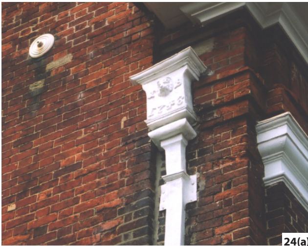
Figure 24: Avoidable loss of a rainwater head: (a) Eighteenth-century original. (b) Inappropriate replacement.
