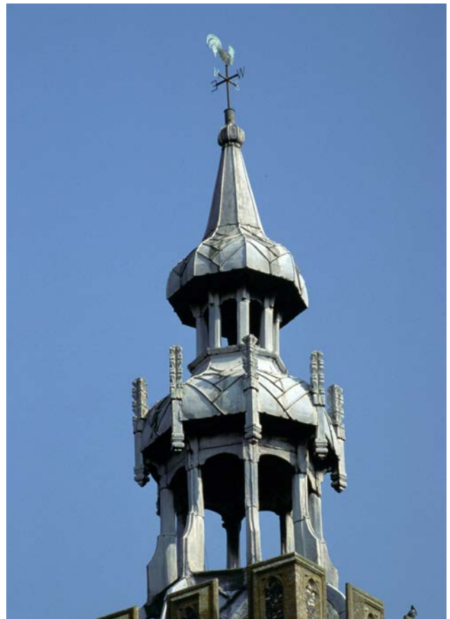
Figure 4: Typical example of a country church flèche at All Saints', Shipdham, Norfolk. Lead was dressed over a complex timber frame to provide a distinctive silhouette to the skyline.
