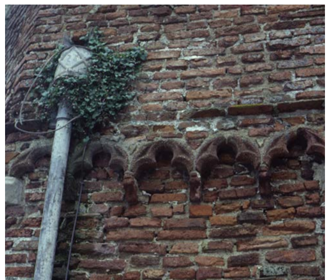
Figure 27: Vegetation growing in lead rainwater head: an obvious problem with a simple remedy.
