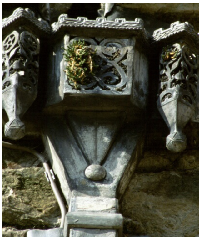
Figure 21: Moss and other organic matter lodged in pierced bartizans, prior to cleaning. Knole, Kent.
