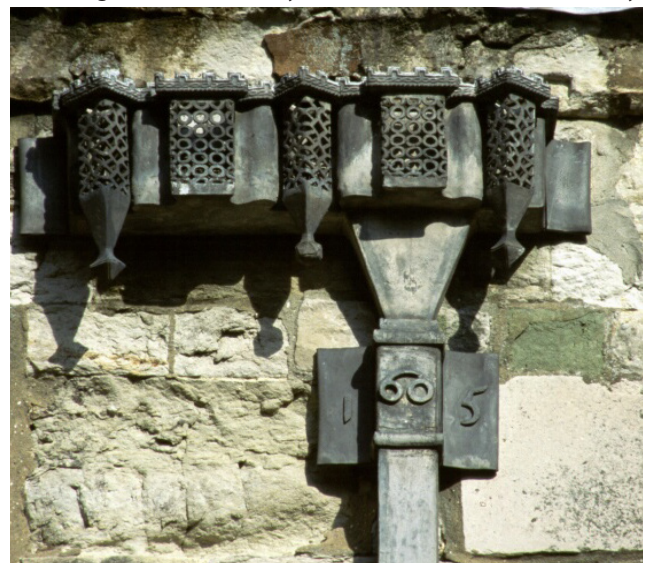
Figure 16: Combination of sheet lead sections shaped over wooden block, soldered and wiped soldered with pierced work added. Note the shadows cast by the solid pendants. Knole, Kent, 1605. Photo: Peter T J Rumley
