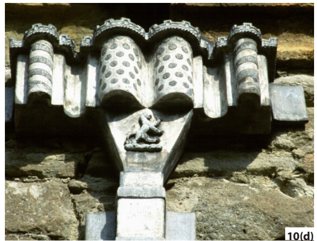
Figure 10: Colourful surface treatment: (a) Gilded rainwater head, Upnor Castle, Kent, 1718. (b) Painted rainwater head, Tilbury Fort, Essex, 1719. (c) Gilded and painted pipe collar, St John's College, Oxford, 1635. (d) Tinning of circles and chevrons, Knole, 1605. Photos: Peter T J Rumley
