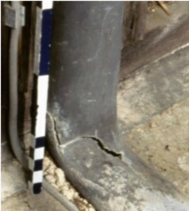
Figure 22: Common failure of a lead soil pipe, prior to repair. Ightham Mote, Kent. Photo: Peter T J Rumley
