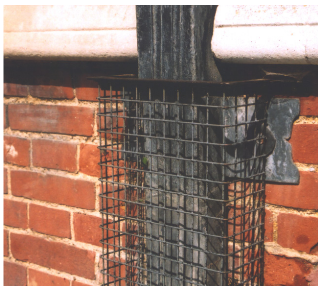
Figure 25: Protection for a decorative lead downpipe. Photo: Douglas Kent
