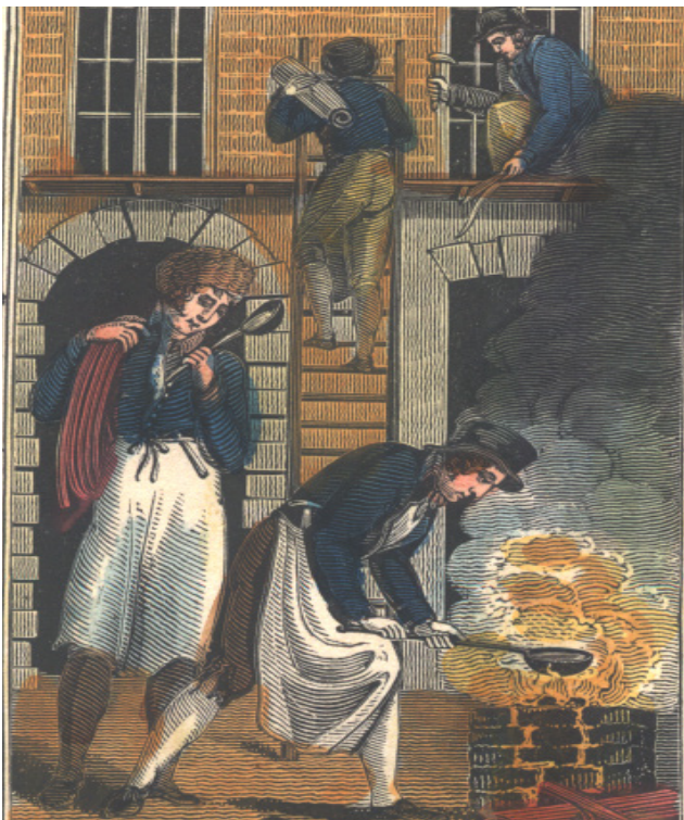
Figure 2: Early 19th-century print (anon) showing plumbers undertaking sheet leadwork. Note the soldering iron in the foreground. Photo: Philip Venning
