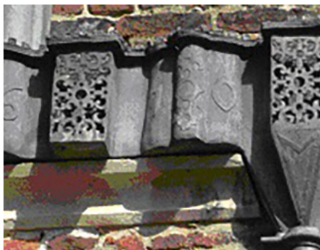
Figure 18: Pierced work with tinning on bartizans, Hatfield House, Hertfordshire, 1610.
