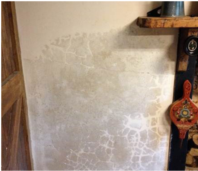
Figure 6: Rising dampness exists but is rarer than commonly supposed. Photo: Caroline Rye
