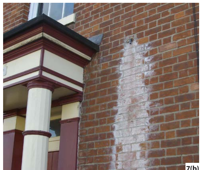
Figure 7: Plumbing leaks associated with: (a) Defective pipework above a kitchen unit (b) Overflowing WC cistern.
