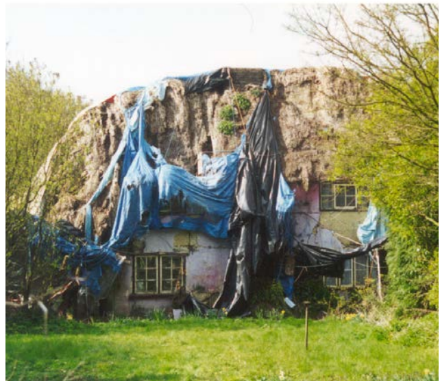
Figure 1: Dampness can lead to serious deterioration if left unattended, as with this cottage that was later demolished as a result. Photo: Douglas Kent
