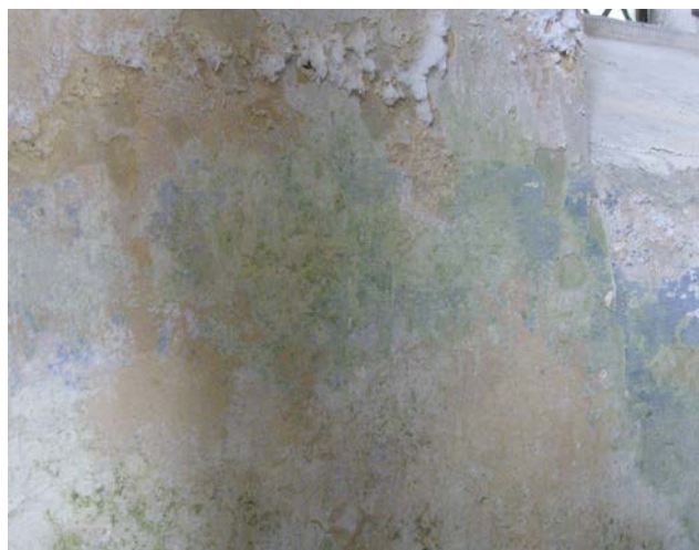
Figure 10: Hygroscopic salt deposits can be a sign of a current or past rising dampness problem.
