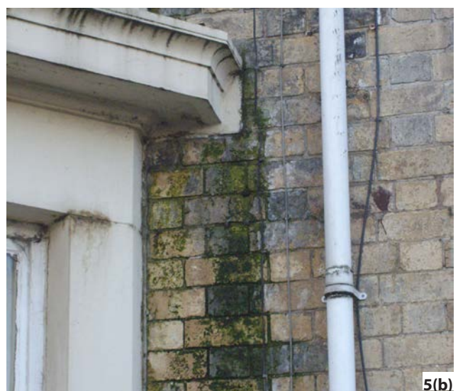
Figures 5: Common symptoms of rainwater penetration. (a) Water staining internally. (b) Green algal growth externally.
