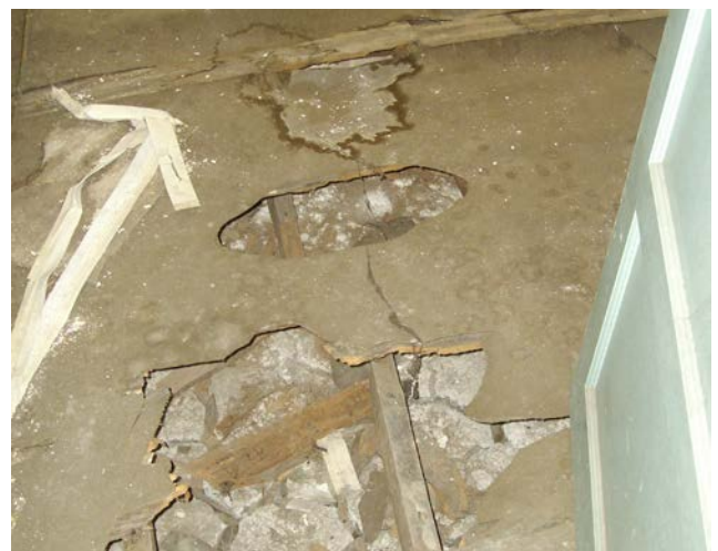
Figure 11: Decay of floor structures can result from high humidity in voids below.
