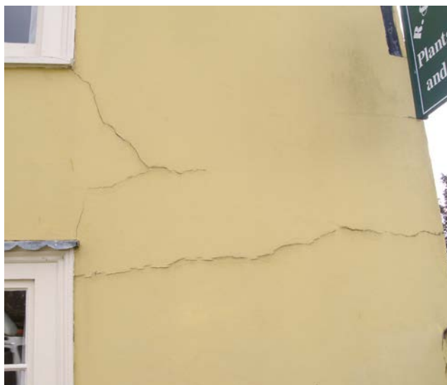
Figure 15: Hairline cracks resulting from the inappropriate use of cement render on traditionally constructed buildings can admit moisture via capillary action. Photo: Douglas Kent
