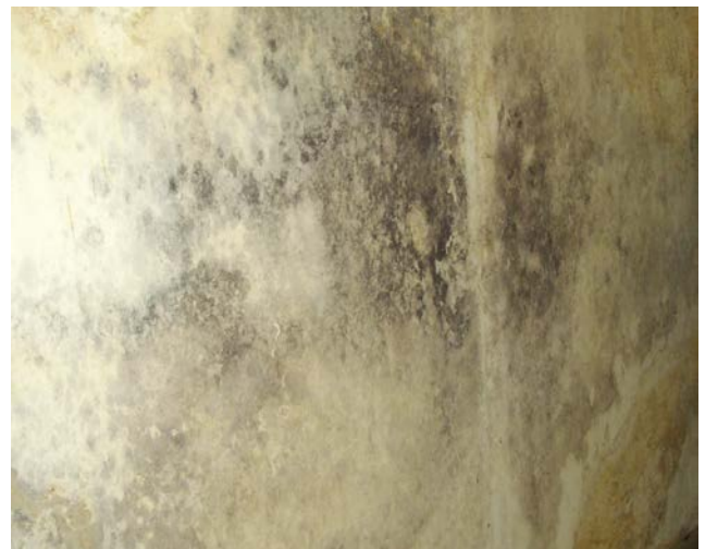
Figure 9: Black spot mould is commonly associated with condensation.
