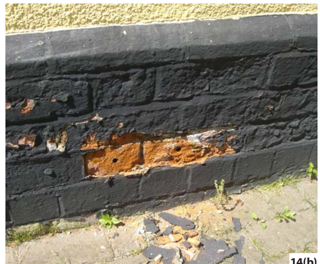
Figure 14: Traditional, solid walls can suffer from dampness and deterioration where inappropriate impermeable finishes are used, such as: (a) Plastic-based paints. (b) Bitumastic products. Photos: Douglas Kent
