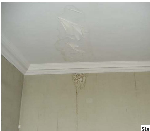
Figures 5: Common symptoms of rainwater penetration. (a) Water staining internally. (b) Green algal growth externally.
