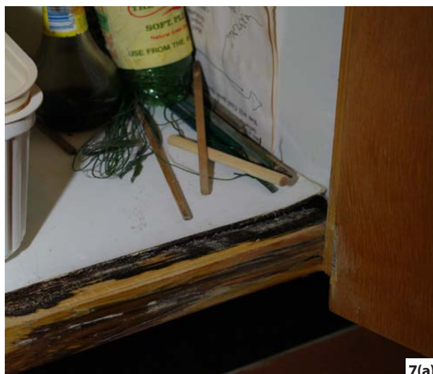
Figure 7: Plumbing leaks associated with: (a) Defective pipework above a kitchen unit (b) Overflowing WC cistern.
