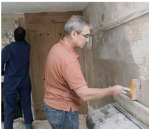
Figure 19: Vapour permeable paints, such as soft distemper, should be used when redecorating traditional solid walls. Photo: Douglas Kent
