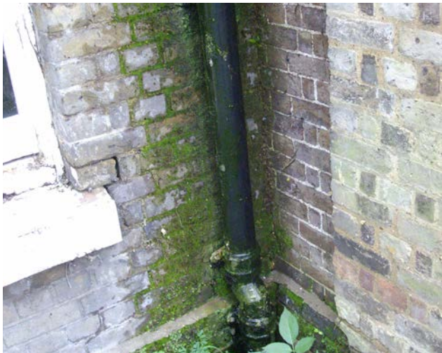
Figure 13: Moss growth can compound problems arising from rainwater penetration. Photo: Douglas Kent
