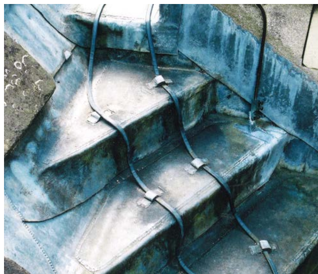
Figure 20: Trace heating cables may be used to prevent the build up of snow and ice in gutters. Photo: Douglas Kent
