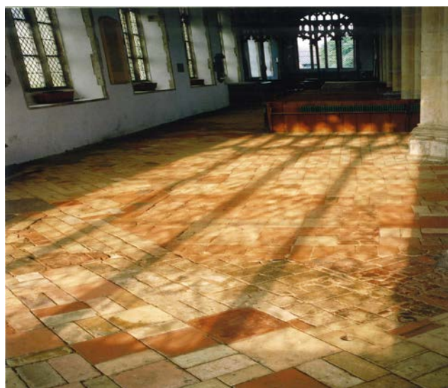
Figure 4: Traditional solid floors allow the ready evaporation of below-ground moisture from their surfaces.
