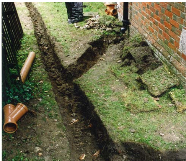
Figure 21: Improvements to drainage can help to overcome problems arising from below-ground dampness.
