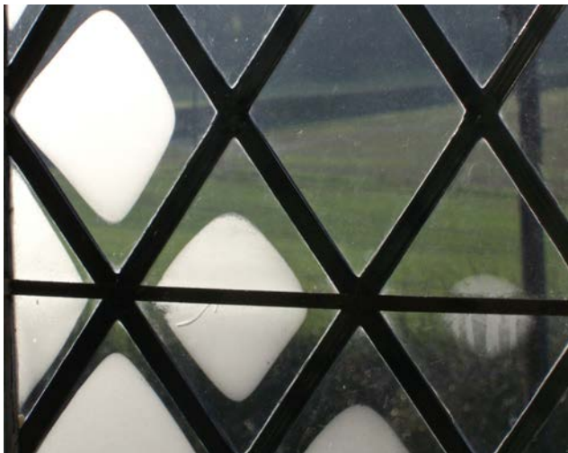
Figure 8: Condensation forms on the coldest surfaces first, such as windows or their surrounding reveals.
