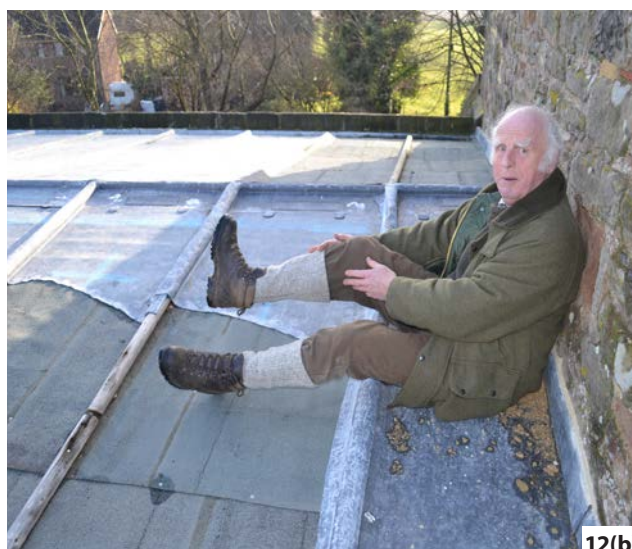
Figure 12: (a) Rainwater penetration due to missing gutter. (b) Damage from lead theft.
