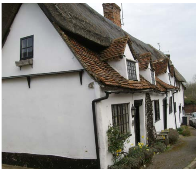
Figure 3: Traditional architectural details, such as pentice boards, function to protect buildings from the rain.
