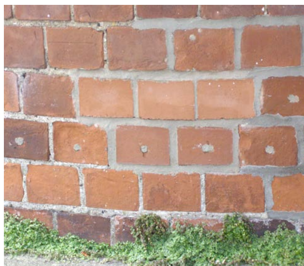
Figure 23: Evidence of holes drilled for chemical DPC injection, which is not only damaging but usually unnecessary in a traditionally constructed building. Photo: Douglas Kent
