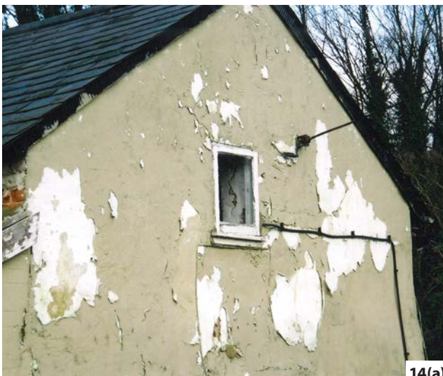
Figure 14: Traditional, solid walls can suffer from dampness and deterioration where inappropriate impermeable finishes are used, such as: (a) Plastic-based paints. (b) Bitumastic products. Photos: Douglas Kent
