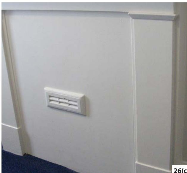
Figure 26: Adequate ventilation helps to prevent condensation, for example, by: (a) opening windows on fine days (b) ensuring subfloor ventilators do not become blocked (c) providing ventilation at the bottom and top of redundant chimney stacks left in place.
