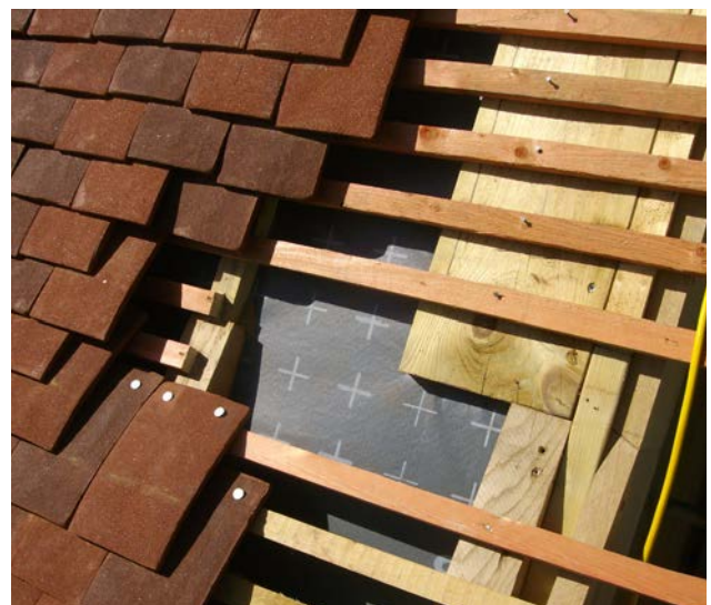
Figure 25: Manufacturers' instructions should be followed closely when installing vapour permeable membranes.
