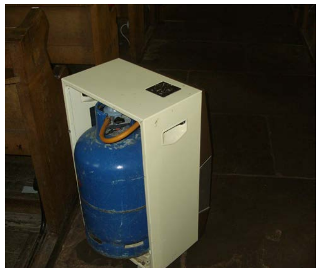
Figure 16: The use of moisture-generating bottled gas heaters is best avoided in thick-walled, solid-floored buildings. Photo: Douglas Kent
