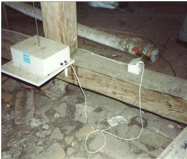
Figure 24: Various damp-proofing systems and dehydration products exist to combat rising dampness. Their use is generally inadvisable on traditionally constructed buildings but where they are installed only those awarded an Agreement or other third-party certificate should be considered.
