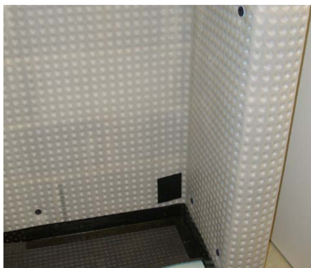
Figure 22: Ventilated dry linings can help with managing below-ground dampness where the underlying cause is difficult to address. Photo: Douglas Kent
