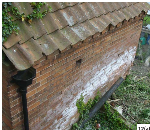
Figure 12: (a) Rainwater penetration due to missing gutter. (b) Damage from lead theft.
