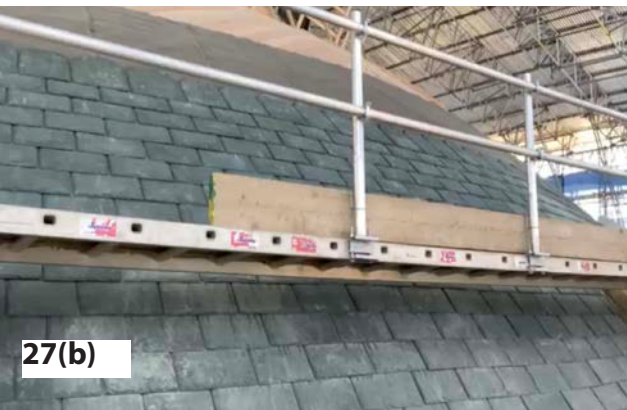
Figure 27. A platform, known as a slater's heel, is used for access on tall roofs provided it can carry the weight of the slater(s) and the slates. It can be a simple scaffold (a). Larger works might justify a more substantial platform using Youngman boards (b).
