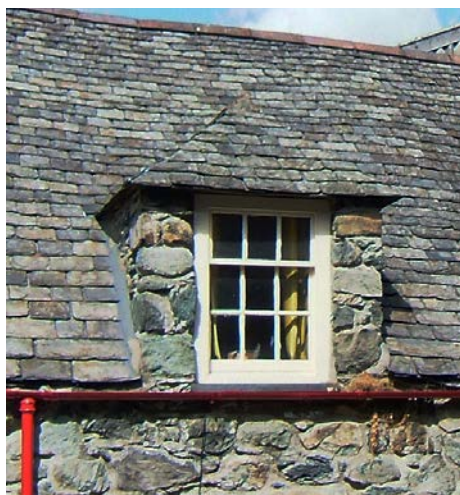
Figure 82. Hipped dormer in Arran Road Dolgellau. Photo Terry Hughes
