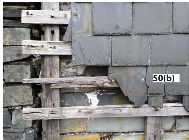
Figure 50. Cladding slates were either pegged into two layers of mortar (a) or peg hung or nailed to battens (b) . Photos Terry Hughes
