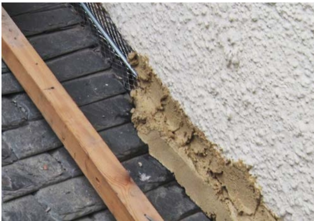
Figure 57. Cracking of mortar fillets can be reduced by incorporating fibre in the mix or with expanded metal reinforcement.
