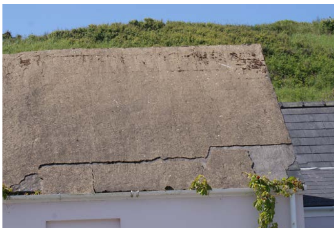
Figure 94. Eventually the weight of slurries overcomes their adhesion, and large sections fall away. Pembrokeshire.
