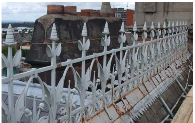
Figure 61 . Cast iron ridge on Chester town hall.
