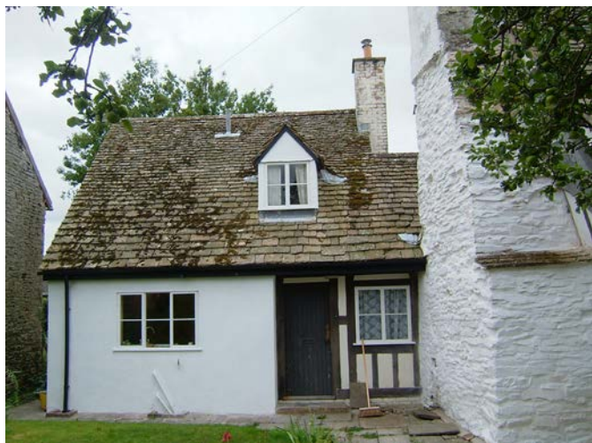
Figure 81. Dormer placed higher in the roof. Colebatch in Shropshire. Photo Terry Hughes
