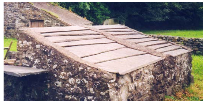
5(b) and (c). In single lap slating each course of slates overlaps only the one immediately below and the vertical sides are butted against each other. Consequently, the perpendicular joints are open and have to be weathered in some other way.
