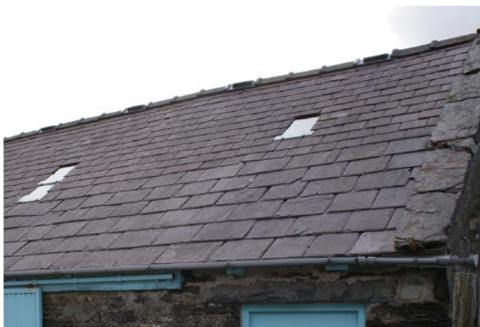
Figure 84. Farm buildings are often lit with sheets of glass which replace slates.
