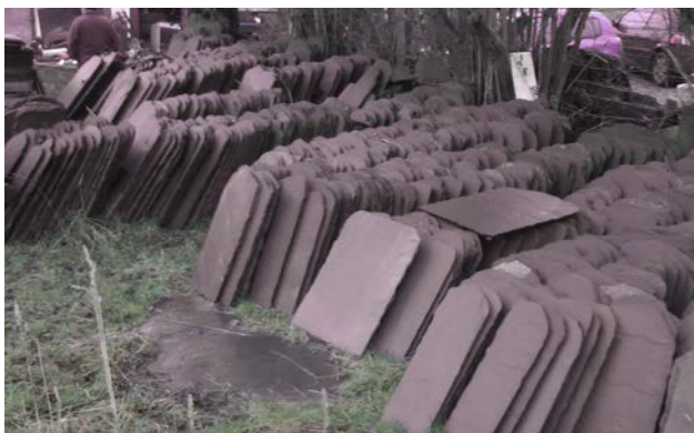
Figure 17. Orders for new slates should not ask for specific sizes. The correct way is to specify the longest and shortest and allow the quarry to produce a natural mix of sizes. It is the slater's job to produce an effective roof from the mix supplied. Hereford stone slates made for St Mary's Church, Portbury, Somerset
