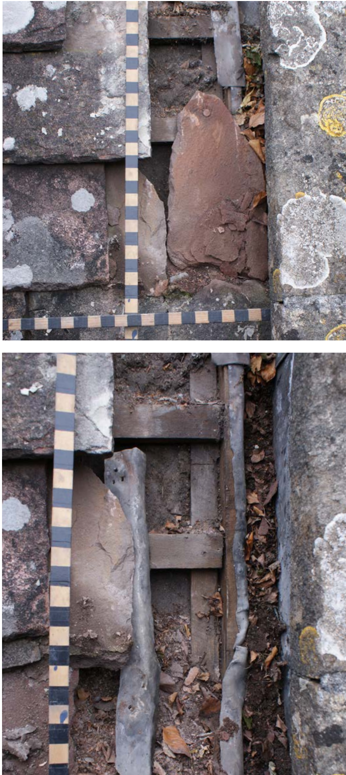
Figure 29. Secret gutters are notorious for becoming blocked by debris. Regular maintenance is essential to prevent leaks Photo Terry Hughes
