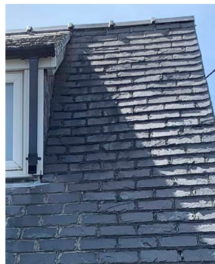
Figure 92. Mastic grouting in an ill-conceived attempt to prevent damp walls. Near Caernarfon. Photo Terry Hughes
