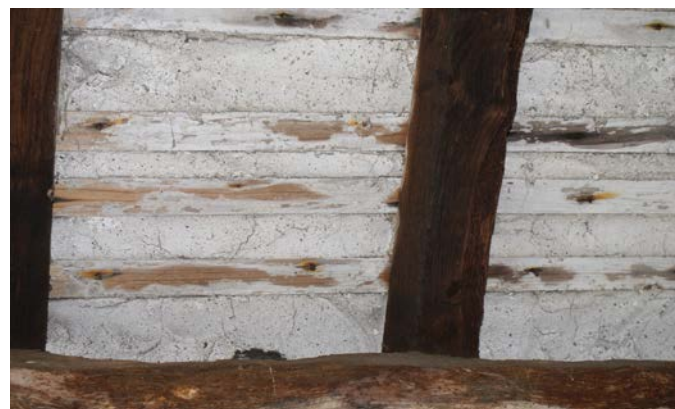
Figure 91. Two coat torching in a cow shed.
