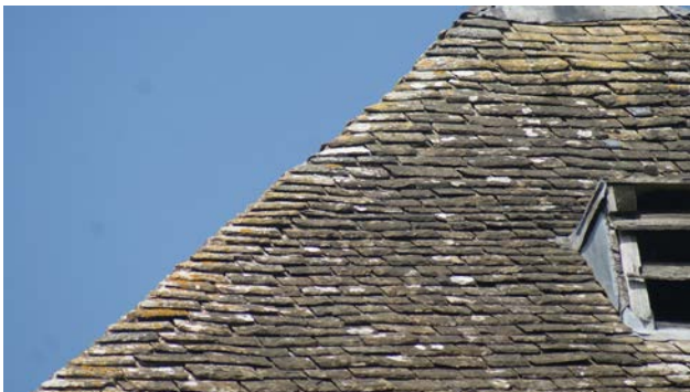
Figure 68. Wide slates are used on mitred hips to reduce the risk of wind damage. Hereford stone on St Mary's church, Kempey
