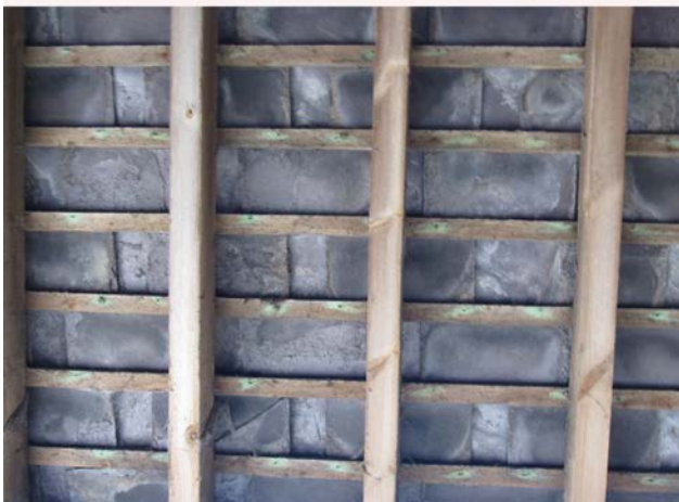
Figure 49. Open slating to provide good ventilation is fairly common on animal housing in the region. Photos Adam Burnett
