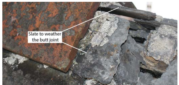
Figure 64. The butt joints of plain ridge tiles were weathered with small slate slips.
