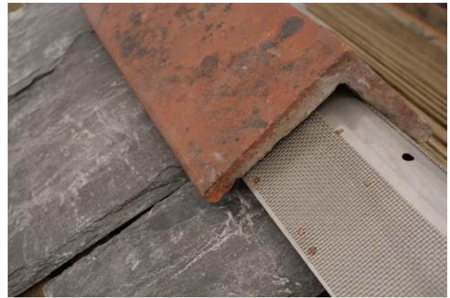
Figure 30. Stainless steel under-ridge vents can be used where it is important to conserve the appearance of the ridge line.
