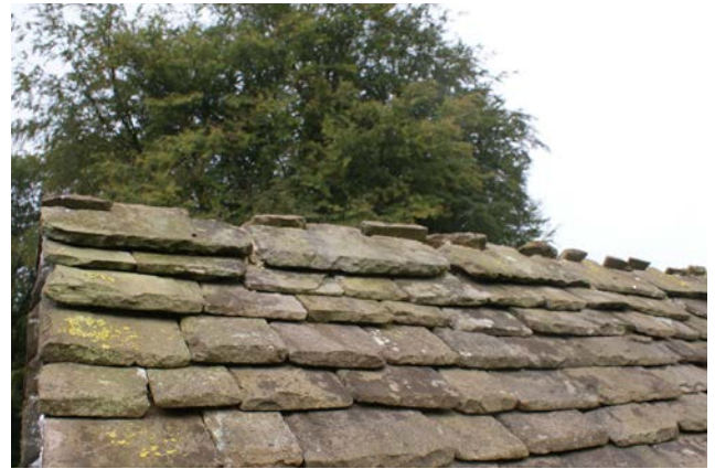
Figure 58. Wrestler ridge on a shed at Kennixton Farmhouse from Llangennith, Gower, Glamorgan. Now at St Fagans museum, Cardiff.
