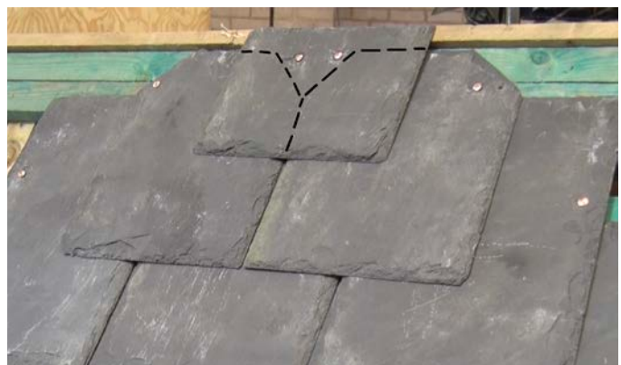
Figure 64. The butt joints of plain ridge tiles were weathered with small slate slips.
