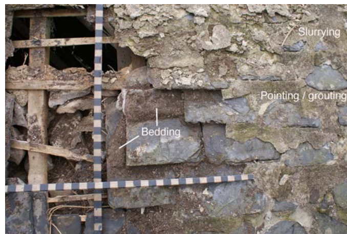
Figure 89. Tail bedding is applied as the slates are laid and should not spread beyond the tail onto the slate below. Pointing, grouting and slurrying are applied long after the slating was laid. Pointing and grouting are spread along the slates tails and forced up under the slate. Slurrying is spread all over the slates. Pembrokeshire.
