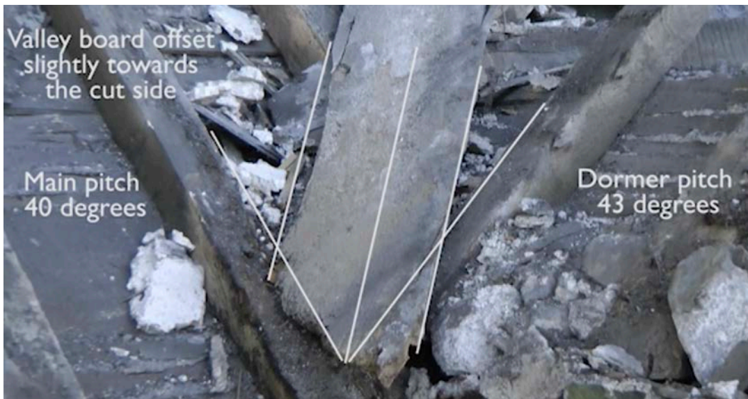
Figure 73. Successful valleys often combine the kill of the joiner (a) and the Figure 66.slater (b). Working together they ensure that water flowing over the slating moves away from the vulnerable junction (c) Photos Terry Hughes
