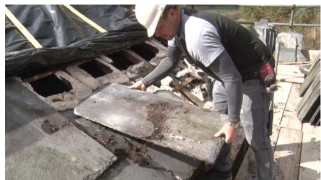
Figure 4. As the major quarries developed and gained access to the deeper, better cleavage slate they were able to make larger slates. These were known as rags, queens or tons. As much as 48" (1.2 m) long they were able to compete with the large sandstones slates of the Pennine counties.
