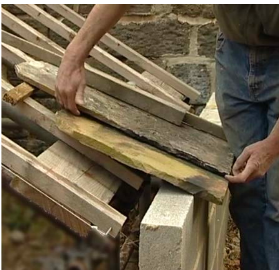
Figure 51. To ensure slates in each course lie closely onto each other the eave is tilted slightly.
