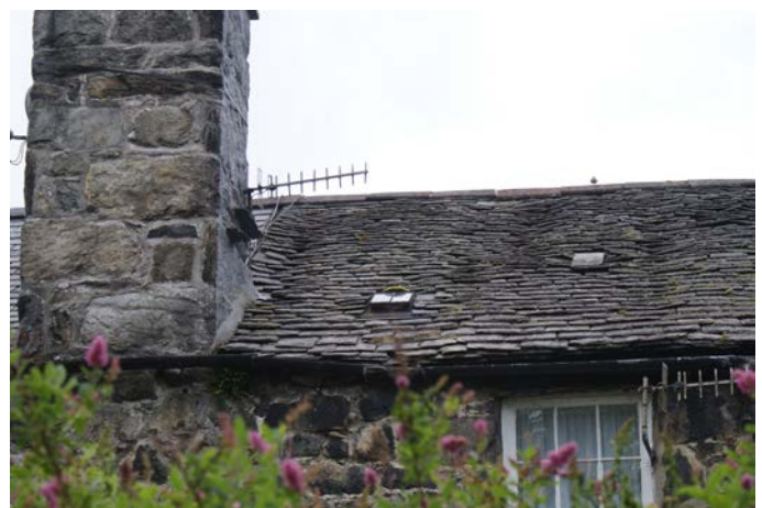
Figure 85. Original rooflights were generally small and low profile, making a small impact on the appearance of the roof.
