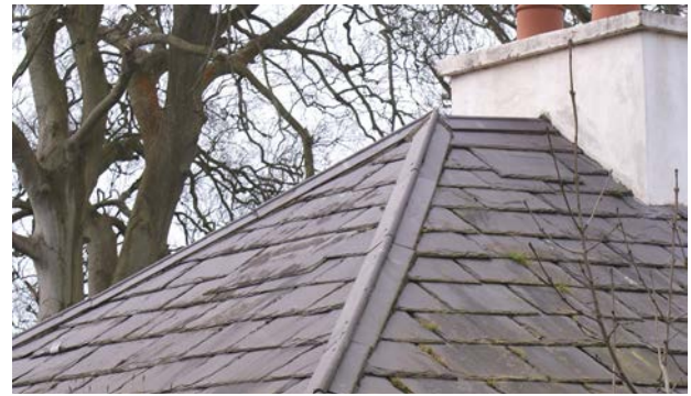
Figure 69. Slate ridges were equally suitable for hips.
