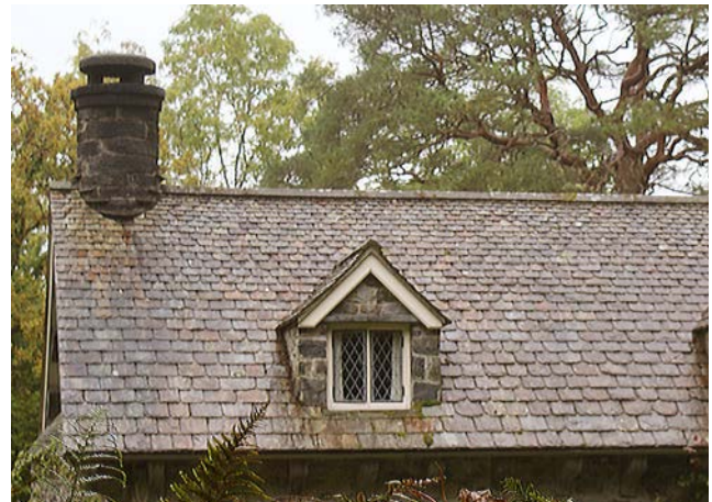
Figure 34. Smaller quarries usually working near-surface slates produced so-called rustic slates which were iron-stained. This example is near Llanrwst, Gwynedd.
