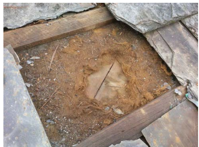
Figure 28. The earliest underlays were based on vegetable fibres or hair and were intended to insulate roofs.
