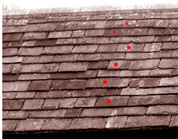
Figure 32. If the batten gauge is not adjusted at change courses, there will be long margins above short ones indicating that the head lap will probably be inadequate.
