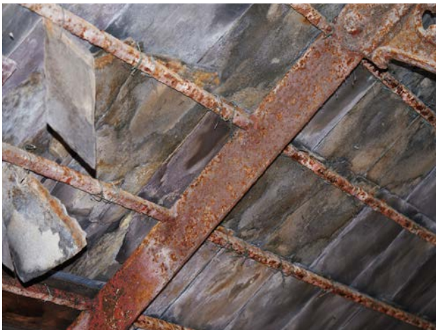
Figure 47. The development of iron framed buildings to resist fires eventually included the roof structure with iron trusses and laths (a). The laths were often set into notches in the rafters (b). This dictated the length of slate which would be used.
