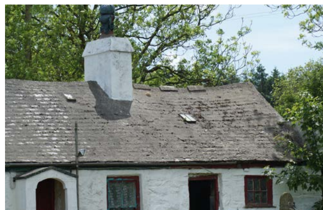
Figure 93. Slurred roof at Rhosgadfan, near Caernarfon. Photos Terry Hughes
