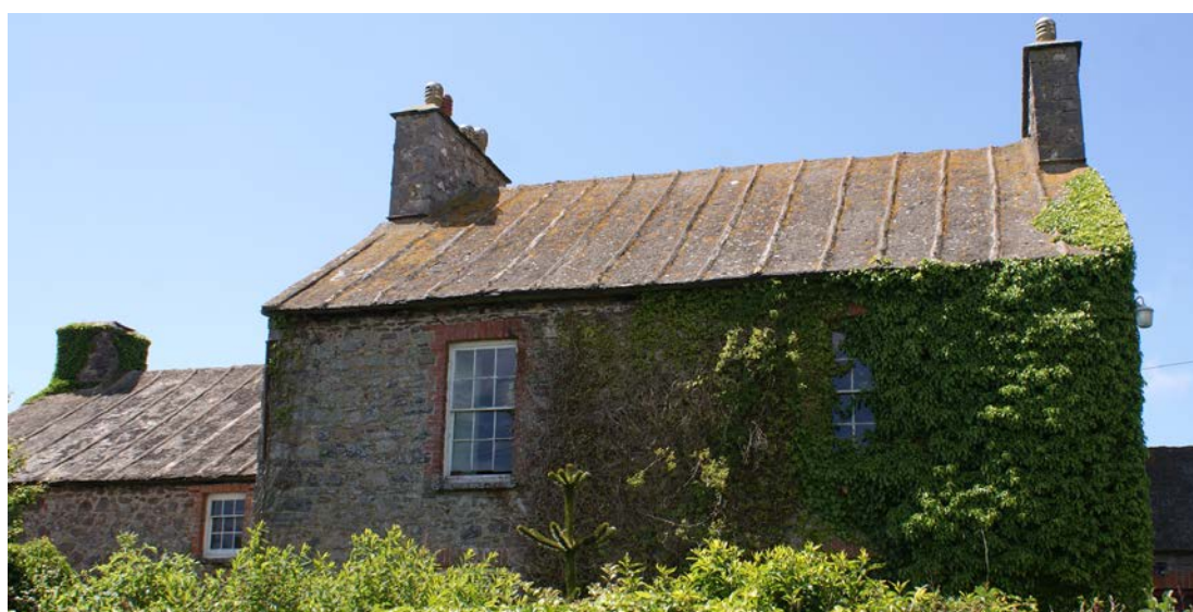
Figure 95. Reinforcing ribs on a Pembrokeshire roof.
