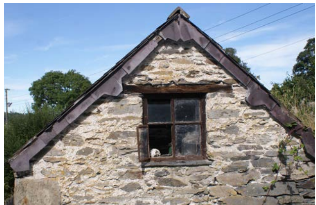
Figure 55. Where an external rafter is installed it is often protected with barge slates.
