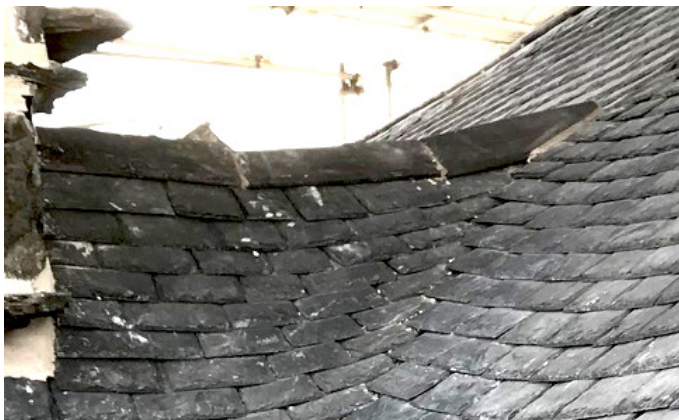
Figure 65. Before the use of lead saddles, the difficult junction between a dormer ridge and the main slope was weathered by sweeping the slates and the ridge up into it.
