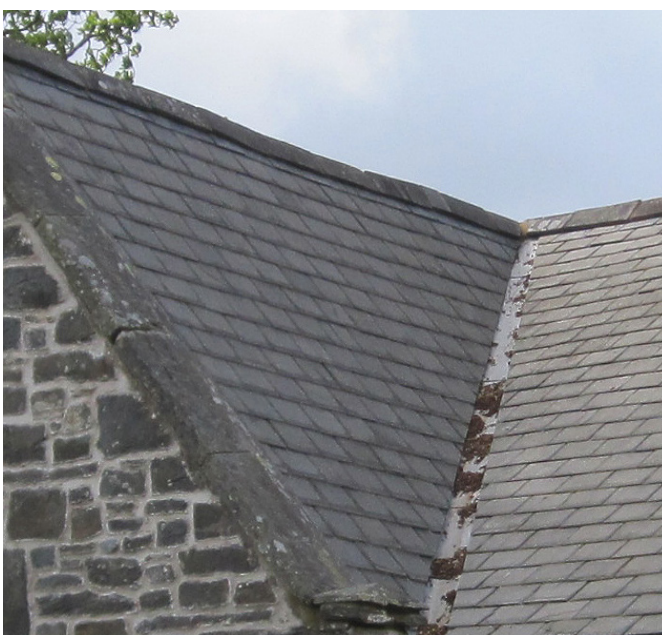
Figures 6 and 7. The Welsh slate valley in the top photo which had been satisfactory for at least 100 years was changed to a lead lined type for no good reason.
