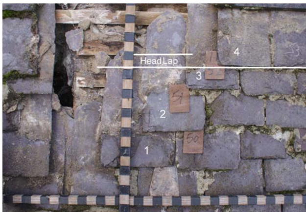
5(d). In triple lap slating the fourth course overlaps the first and so on. This makes it possible to use slates which would be too narrow for double lap slating without risking leaks. It also improves the wind resistance. Less common in Wales than in south-west England, it has been identified only on a few roofs so far.
