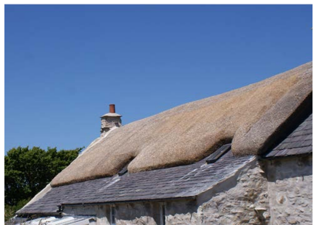
Figure 22. Slates below thatch. Roson farm, Pembrokeshire. Photo Terry Hughes
