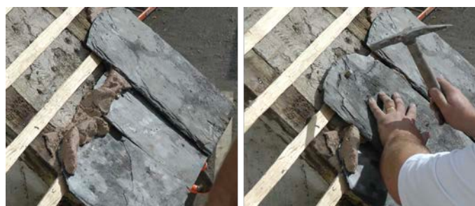
Figure 90. Head bedding is applied as the slates are laid.
