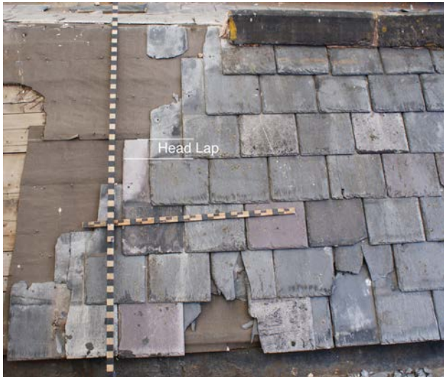
5(a). In double lap slating the third course overlaps the first, fourth overlaps the second and so on, usually by a specified amount - the head lap. This is how all new and many old roofs are constructed. (Ditherington Flax Mill, Shropshire).
