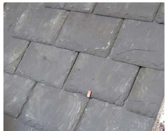
Figure 19. Slipped slates can be refixed with a tingle. Copper is better than lead, which tends to unroll.
