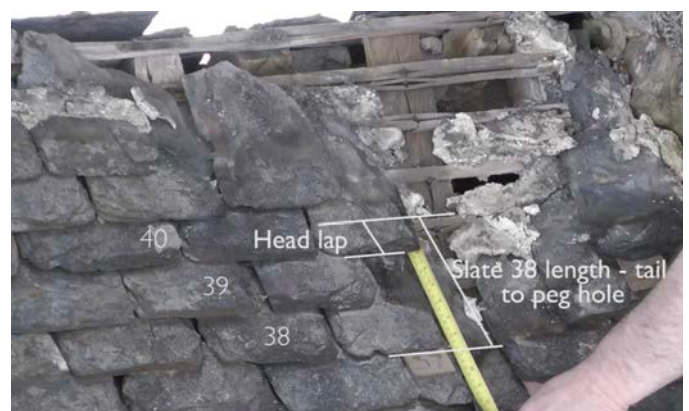
5(e). A system of slating in thirds where the head lap and the lath gauge are equal to the slate length (from tail to peg hole) divided by three. The method uses a divider rather than mathematical division, similar to the techniques of mediaeval masons (video 1).
