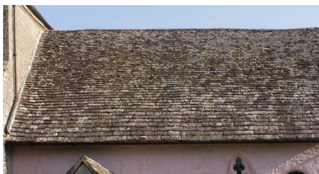
Figure 16. The appearance of slate and stone roofs depends on the mix of sizes which the quarry can produce. St Mary's Church, Kempeley, Gloucestershire
