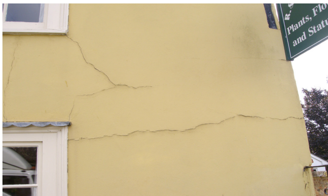
Figure 15: Hairline cracks resulting from the inappropriate use of cement render on traditionally constructed buildings can admit moisture via capillary action. Photo: Douglas Kent
