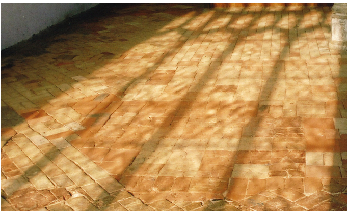
Figure 4: Traditional solid floors allow the ready evaporation of below-ground moisture from their surfaces. Photograph: Douglas Kent
