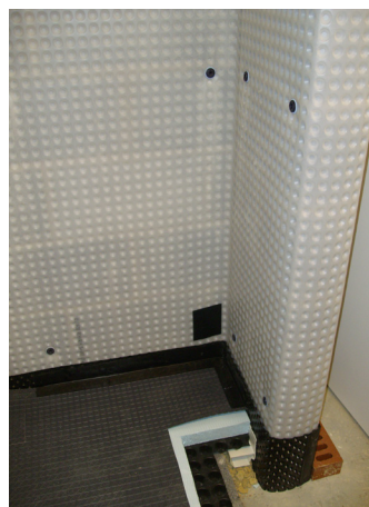
Figure 22: Ventilated dry linings can help with managing below-ground dampness where the underlying cause is difficult to address. Photo: Douglas Kent
