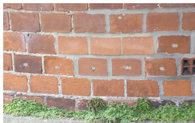
Figure 23: Evidence of holes drilled for chemical DPC injection, which is not only damaging but usually unnecessary in a traditionally constructed building. Photo: Douglas Kent
