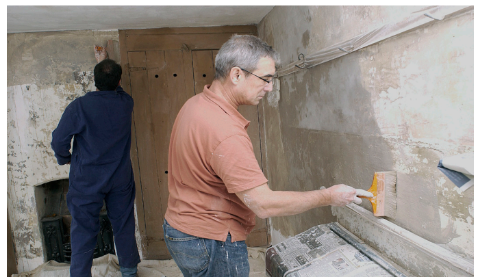
Figure 19: Vapour permeable paints, such as soft distemper, should be used when redecorating traditional solid walls. Photo: Douglas Kent
