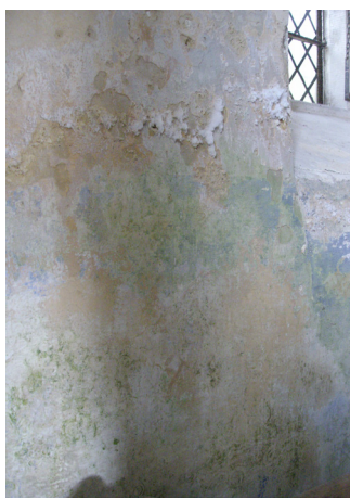
Figure 10: Hygroscopic salt deposits can be a sign of a current or past rising dampness problem. Photo: Douglas Kent
