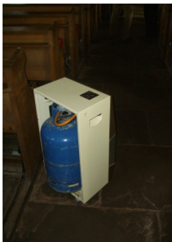
Figure 16: The use of moisture-generating bottled gas heaters is best avoided in thick-walled, solid-floored buildings. Photo: Douglas Kent
