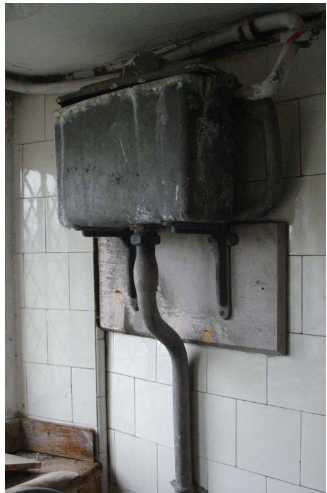
Figure 1: Lead water pipe for WC with wiped soldered joint below cistern. Photo: Douglas D Kent
