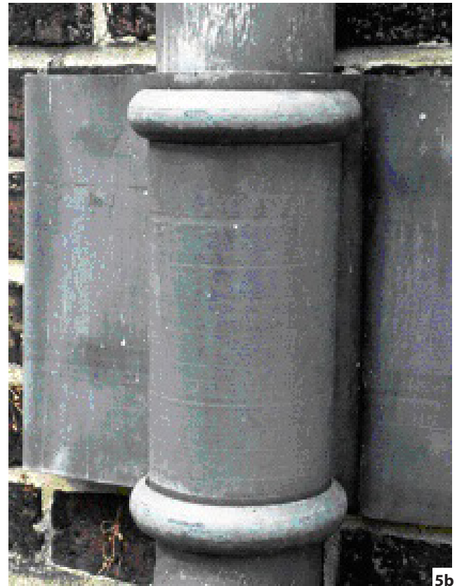
Figure 5: Collars: (a) Early 'false' collar and spigot joint formed simply by opening and closing the ends of the lower and upper pipes respectively, and applying cast astragals to the lower pipe, along with a band to create ears for fixing to the wall.
