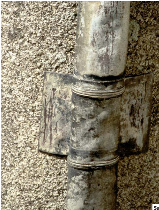
Figure 5: Collars: (a) Early 'false' collar and spigot joint formed simply by opening and closing the ends of the lower and upper pipes respectively, and applying cast astragals to the lower pipe, along with a band to create ears for fixing to the wall.
