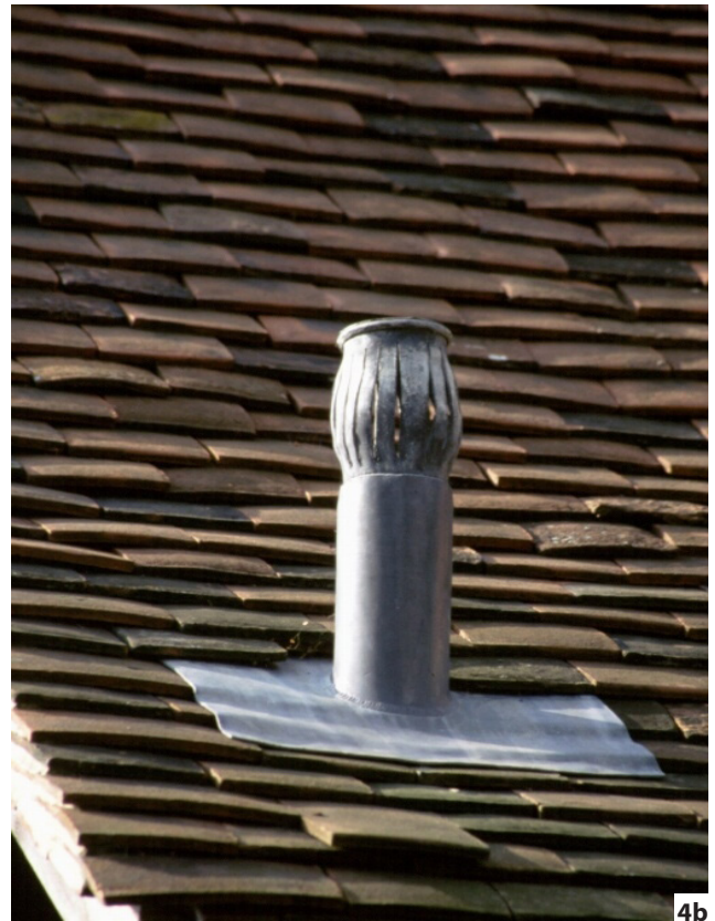
Figure 4: Lead drainage pipes: (a) Rainwater and waste water disposal. (b) For air venting, incorporating roof flashing.
