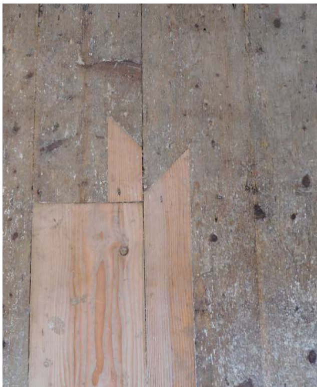
Figure 5: Patches of same timber variety and matching grain. Photo: Philip Hughes
