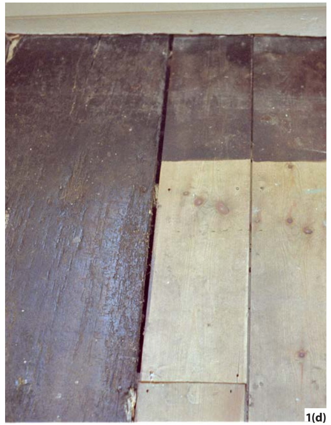
Figure 1: Damage to boards caused by: (a) and (b) Careless lifting and relaying during installation of central heating and wiring runs. (c) A castor, which can be particularly serious when the castor is positioned over the edge of a board. Softwood boards have been used inappropriately in (d) to replace a damaged wide elm board – could it have not been repaired? Photos: Philip Hughes
