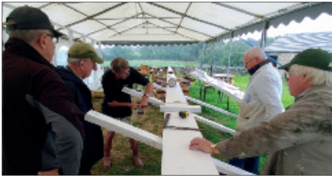
Fitting one of the sail arms into its mortise in the stock.
