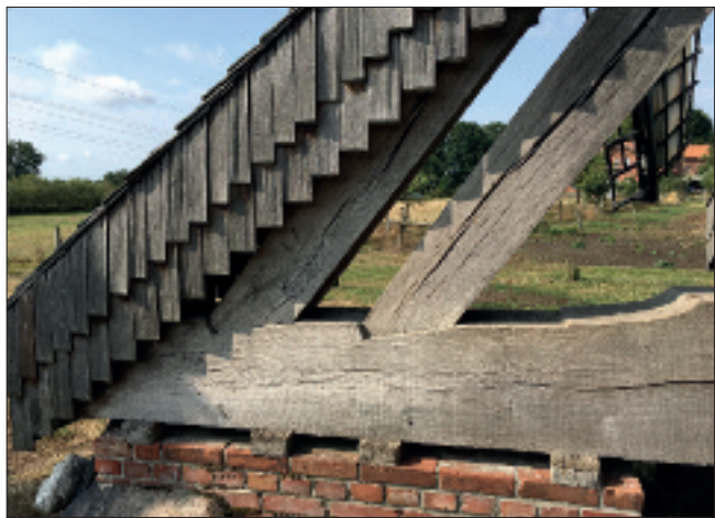
Dudensen mill showing shingle-covered quarterbars.
