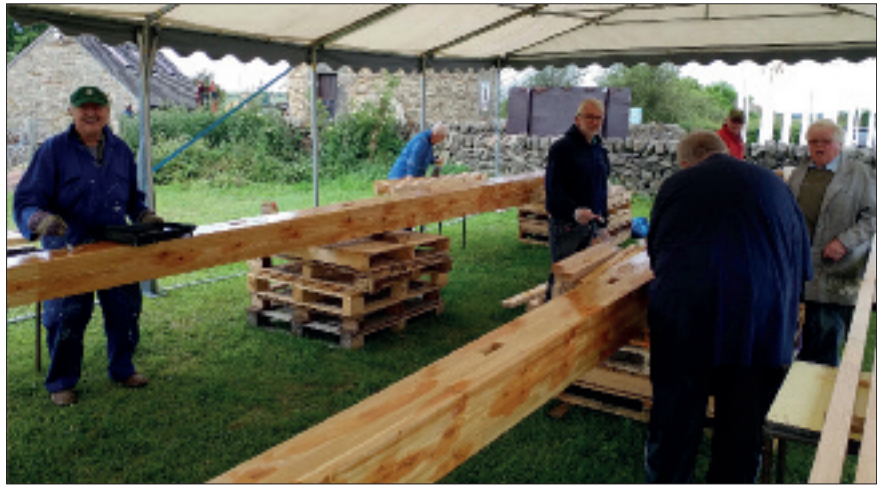
Applying sealant to the 'as received' bare wood.
