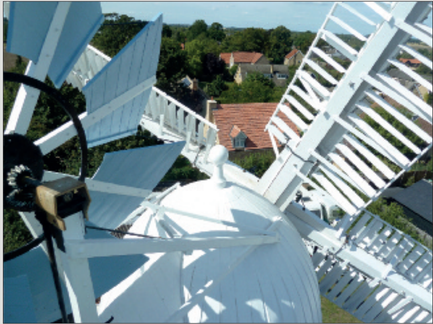
Wicken Windmill photographed from a hydraulic lifting platform in June 2019 while painting and other maintenance work was being carried out on the sails, cap and fantail.
