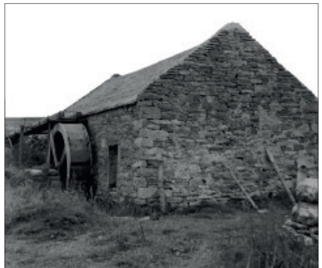
Red House Eday in 1973 – a wooden waterwheeled farm mill. Picture – Peter Burges.
