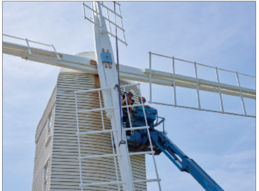
Attaching a sail to the stock at Saxted Mill. Picture – Cbris Ridley, English Heritage.
