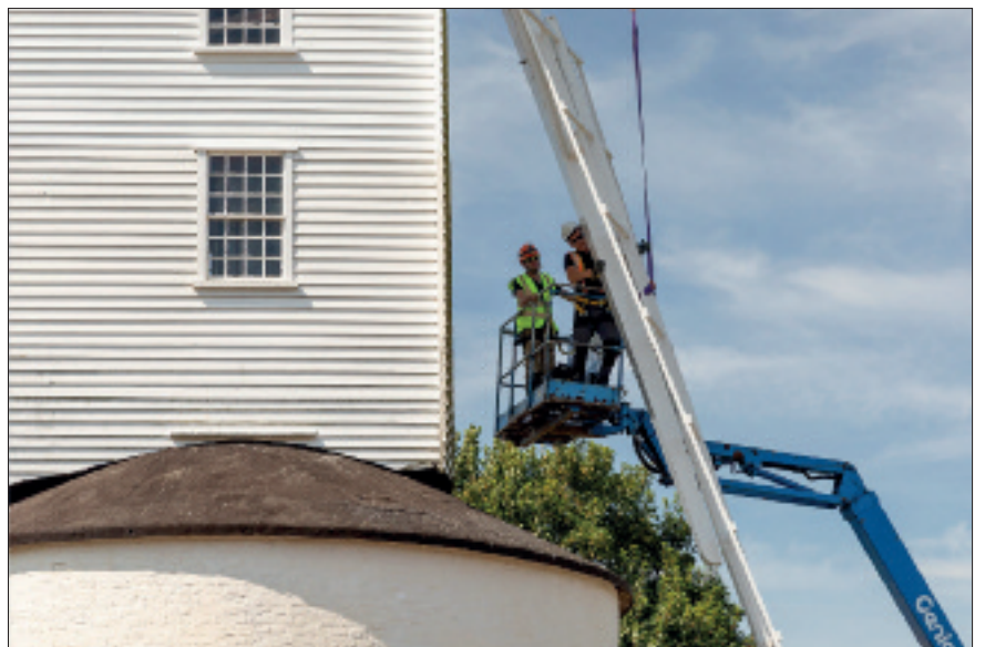
Steadying a sail as it is lifted at Saxstead Mill. Picture – Justin Minns.
