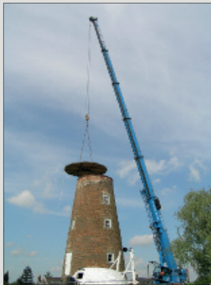
Placing the temporary cap on Billingsford Windmill and the mill with the cap back in place.
