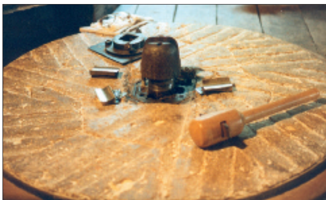
Bedstone spindle being repacked.
