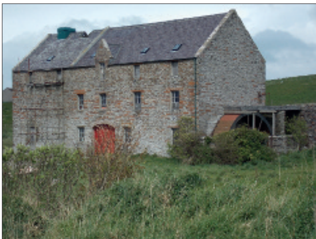
Shapinsay Mill in 2019. Picture – Duncan Hutt.
