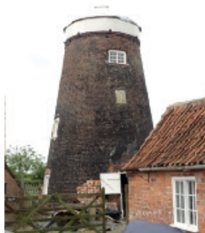
External view of the mill as conserved, with temporary cap.
