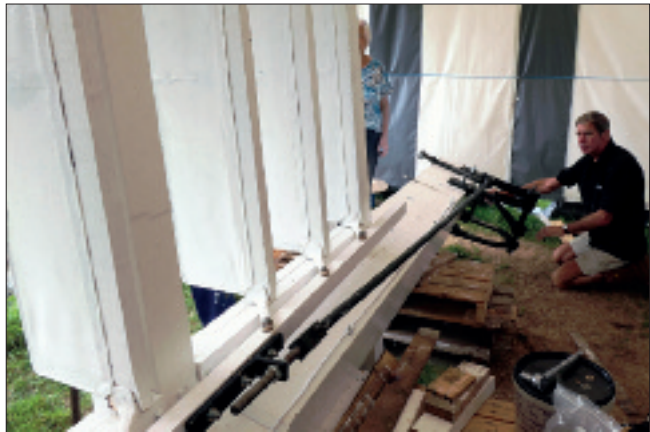
David Land checking the shutter operating mechanism.
