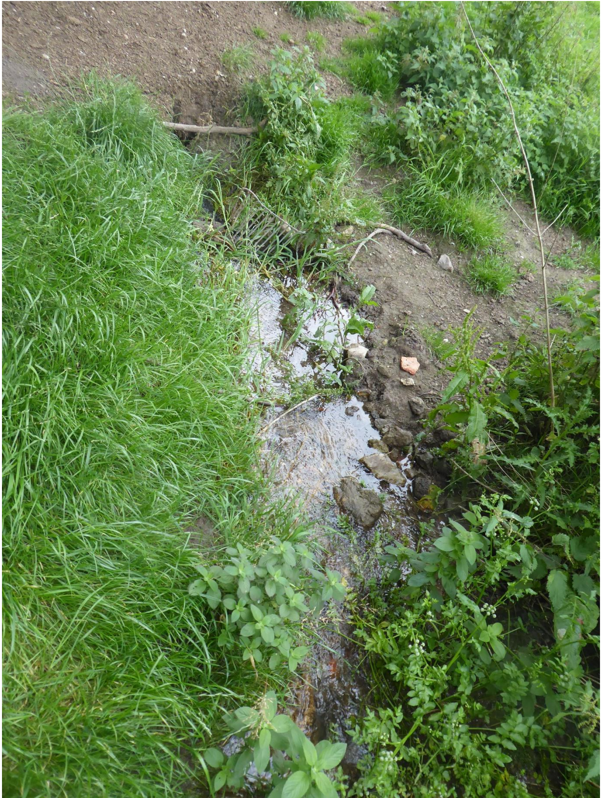
Entrance to culvert at WDC 2
