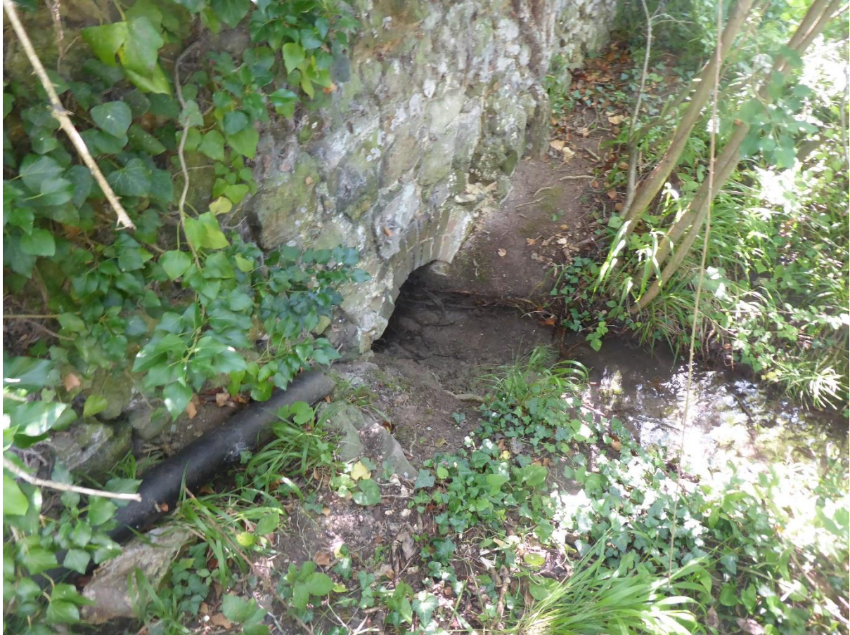
The inlet running under the abbey walls at NP 1.
