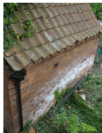
Figure 12(a): Rainwater penetration due to missing gutter. Photo: Douglas Kent
