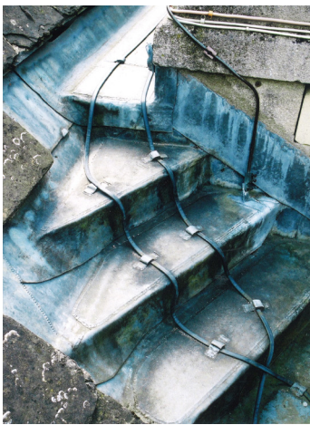
Figure 20: Trace heating cables may be used to prevent the build up of snow and ice in gutters. Photo: Douglas Kent
