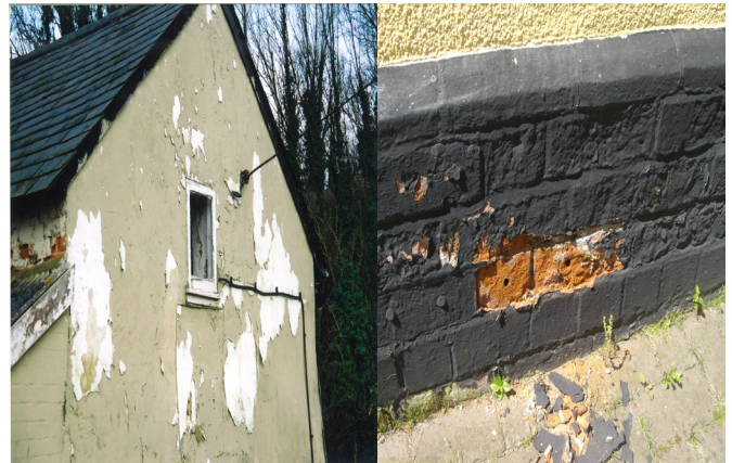
Figures 14(a) and 14(b): Traditional, solid walls can suffer from dampness and deterioration where inappropriate impermeable finishes are used, such as: (a) Plastic-based paints (b) Bitumastic products. Photos: Douglas Kent
