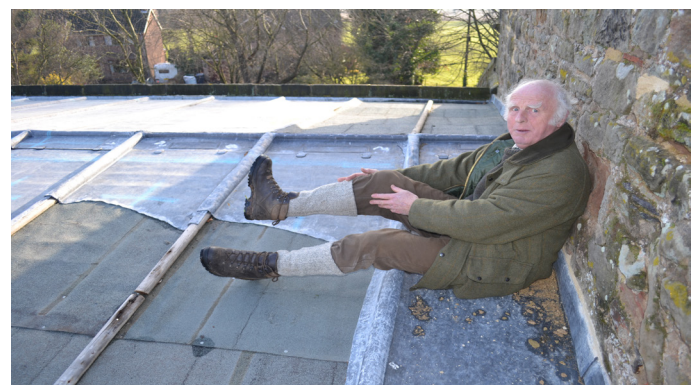
Figure 12(b): Damage from lead theft. Photo: Douglas Kent
