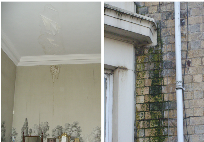
Figures 5(a) and 5(b): Common symptoms of rainwater penetration. (5a) Water staining internally (5b) Green algal growth externally. Photos: Douglas Kent
