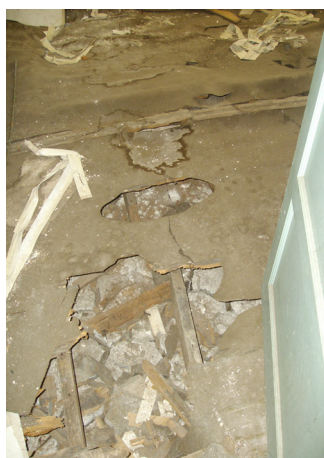
Figure 11: Decay of floor structures can result from high humidity in voids below. Photo: Douglas Kent
