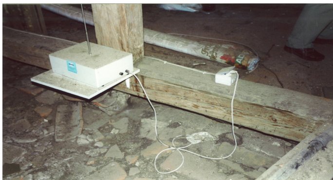
Figure 24: Various damp-proofing systems and dehydration products exist to combat rising dampness. Their use is generally inadvisable on traditionally constructed buildings but where they are installed only those awarded an Agreement or other third-party certificate should be considered. Photo: Douglas Kent
