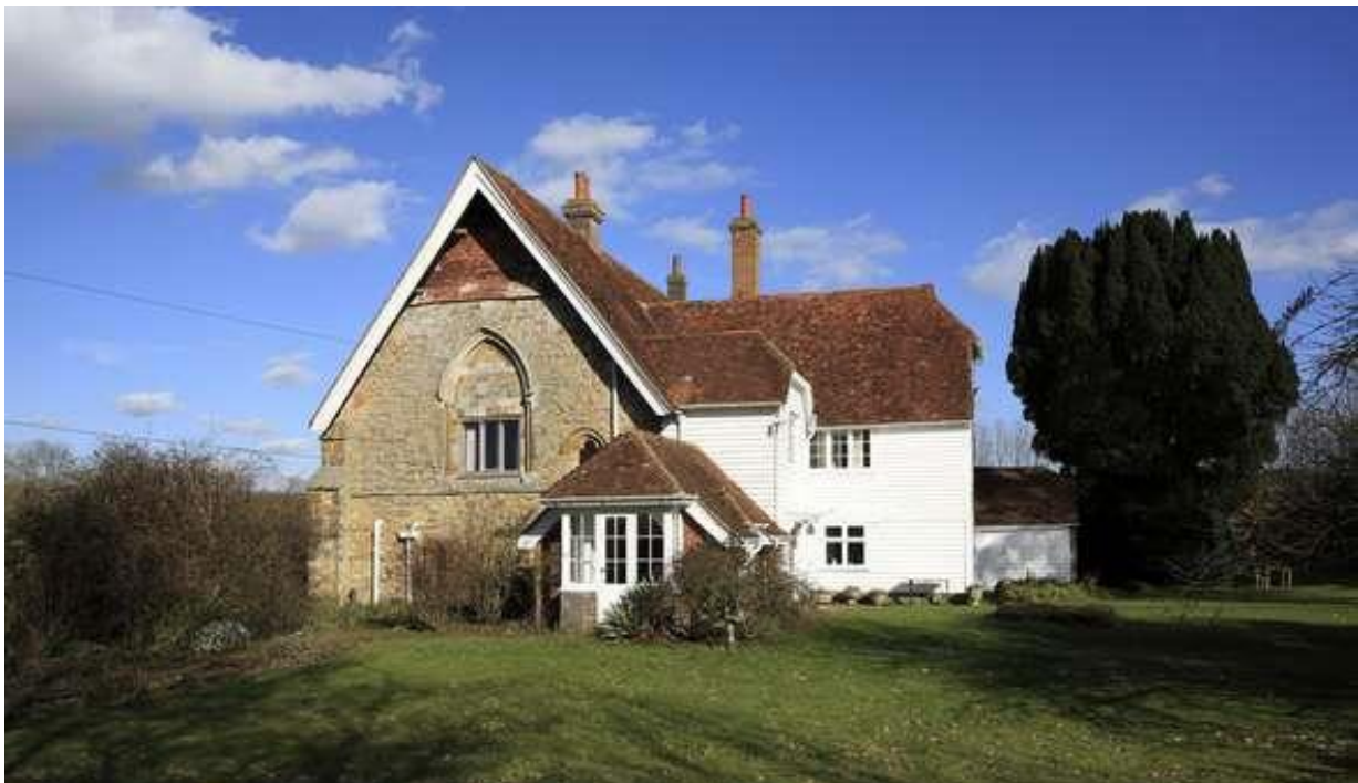
Figure 26 - Abbot's guest hall at the Cistercian Abbey of St Mary's, Robertsbridge, East Sussex. The wooden extension to the right and the porch are modern 'add ons' (Cornwell & Cornwell May 2013).
