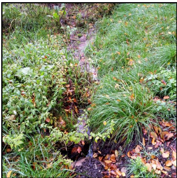
Figure 40 - Boxley Abbey Field A stream entering the culverts at TQ 76086 58745.
