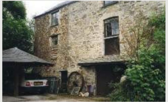
The mill in July 1999. Picture – Martin Bodman.
