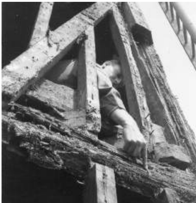
Restoration work on Union Mill, Cranbrook, 1958.
