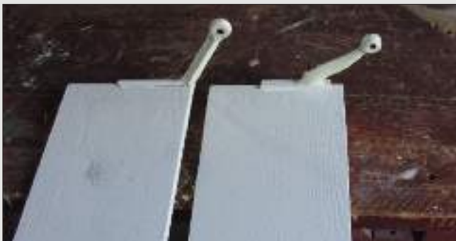
Oldland Windmill, comparison of shutter crank forms.
