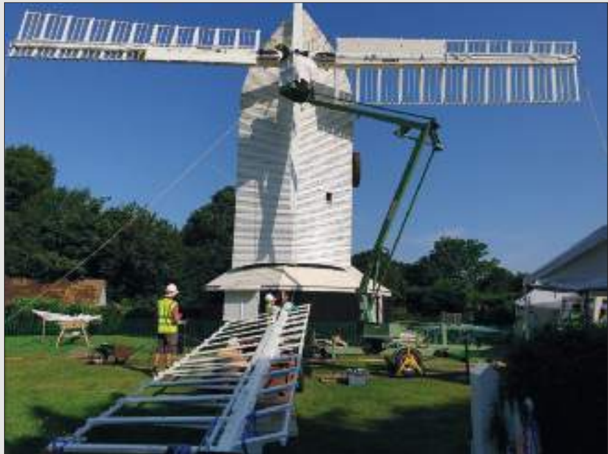
Removing the sweeps at Oldland Windmill.
