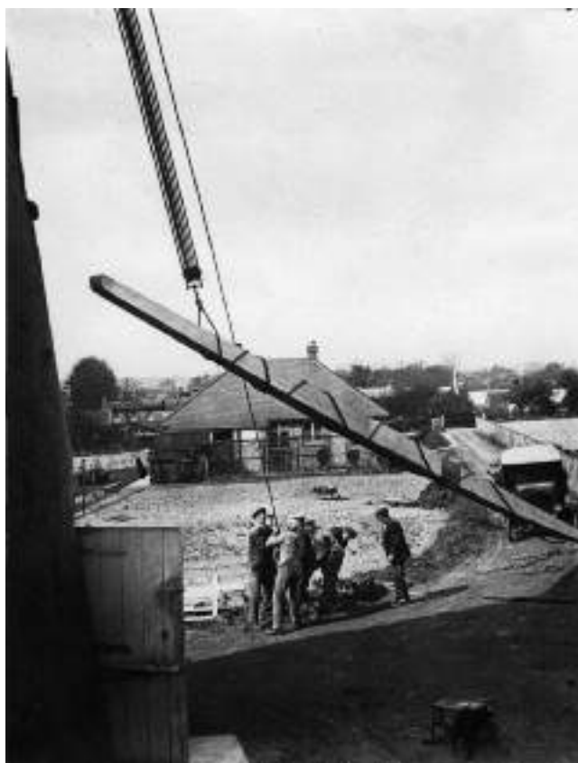
Millwrights at work at Burwell. Picture – Douglas Gavin Reid
