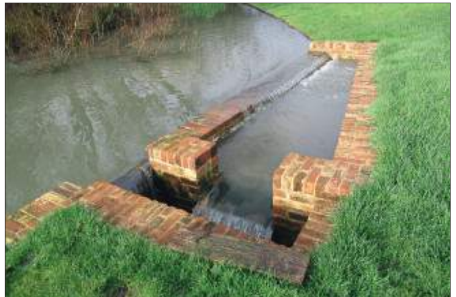
The spillway in the mill pond regulates the water flow with a clever sloping cill. The excess water runs off into the bypass channel, which can be seen on the right of the picture at the start of the article.
