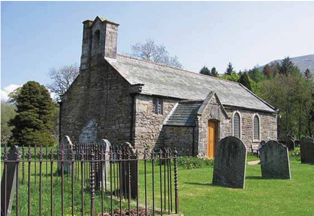
Left, St Mary's, Mallerstang. The SPAB is concerned that proposals for an extension to this ancient building would nearly double its size, and spoil its traditional setting.
